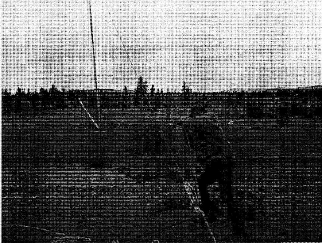
Figure 2.9: Winching a tower into the upright position. This is a 30-m tubular tower being installed at Aishihik Lake (Site # 23). Taller towers require high-power portable electric winches.
