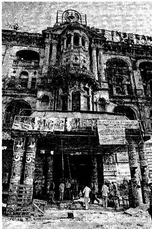
Figure 7.5: Exterior of the Metropolitan Building from Jawaharlal Nehru Road, February 2004. Photo by Author.
