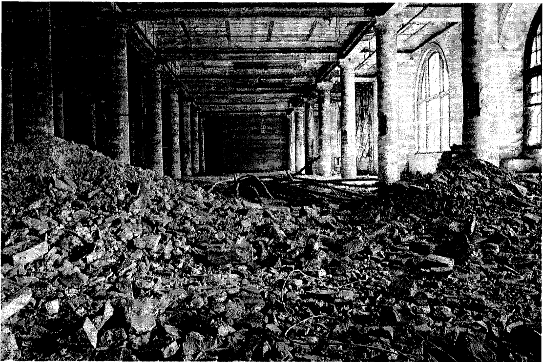
Figure 7.26: Debris piles, interior. February 2004. Photo by Author.
