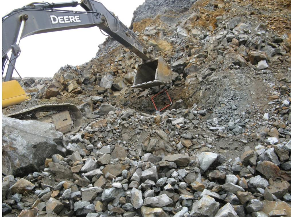
**Photo 2 – Excavated face showing grey traffic surface with oxidized waste rock above**
