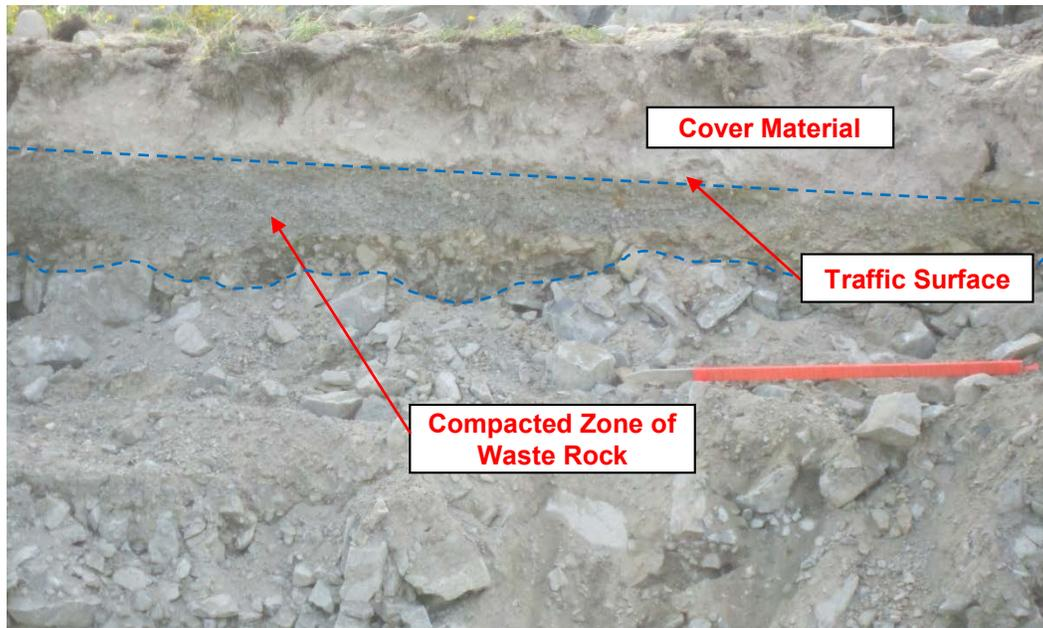
**Figure 4.4 - Waste rock profile showing cover material with underlying traffic surface and zone of compacted waste rock**
