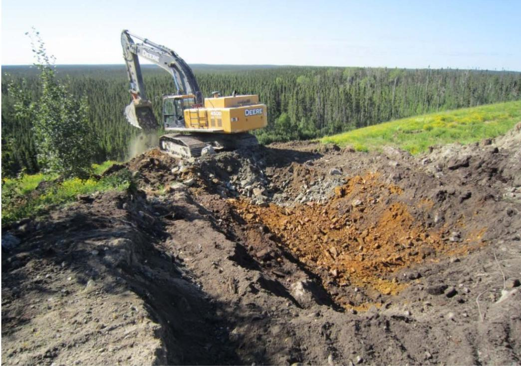
**Figure 3.2 - Backhoe beginning construction of a test pit on WRS 1**
