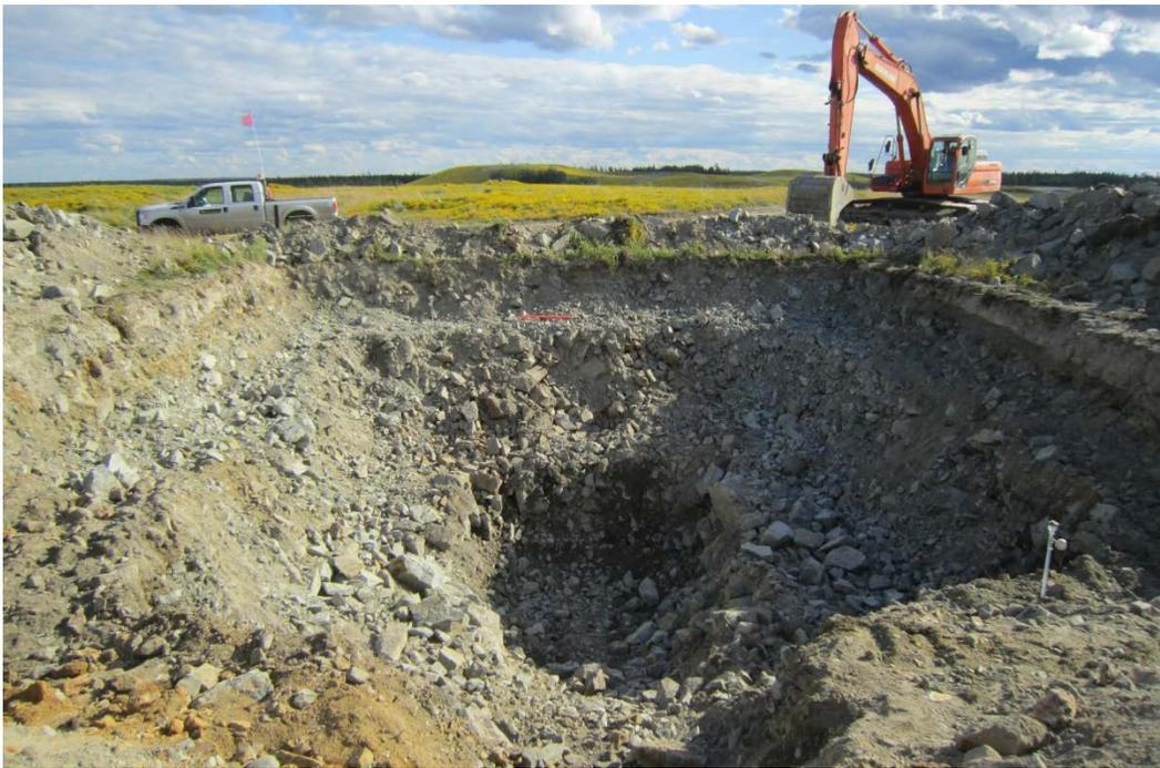
**Figure 3.3 – A typical completed test pit on WRS 2 with tensiometers installed**
