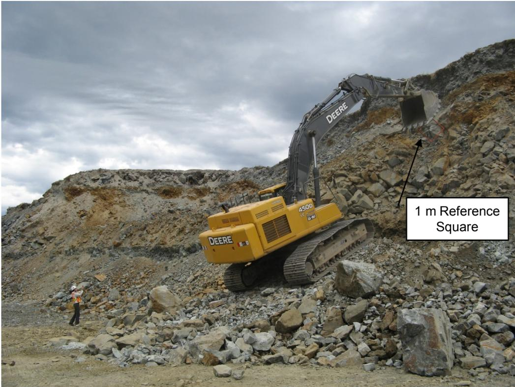
**Figure 3.9 – Profile investigation on Waste Rock Stockpile 1 using an excavator. Note the person for scale and excavator holding reference square for photos taken.**
