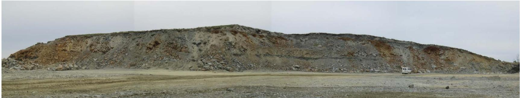
**Figure 4.14 – Excavated North-South face of WRS 1 showing internal structure and variability of oxidation**
