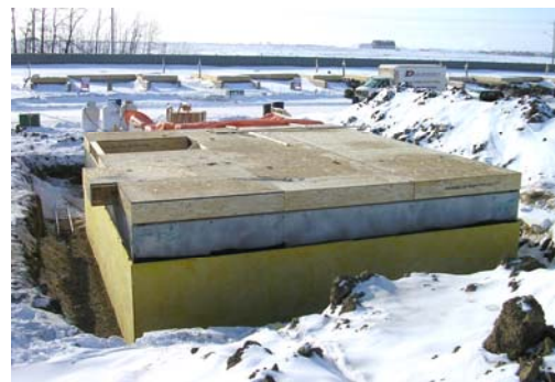
b. Completed PCF Basement
