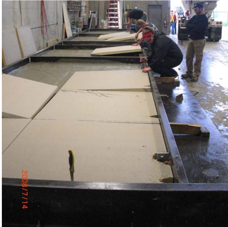
Figure 5-9: Working Bed for Sandwich Panels
