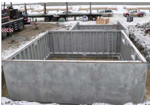
a. Erected Precast Concrete Foundation
