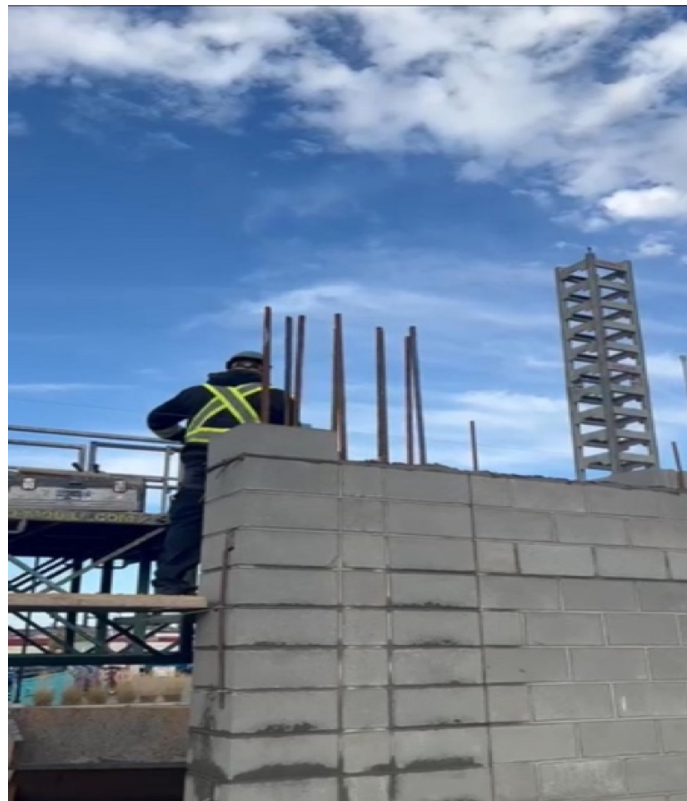
Figure 9: Wall Being Built.
