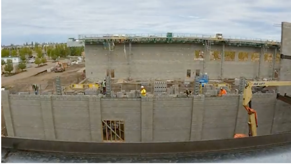
Figure 10: View of Wall Section Being Built.
