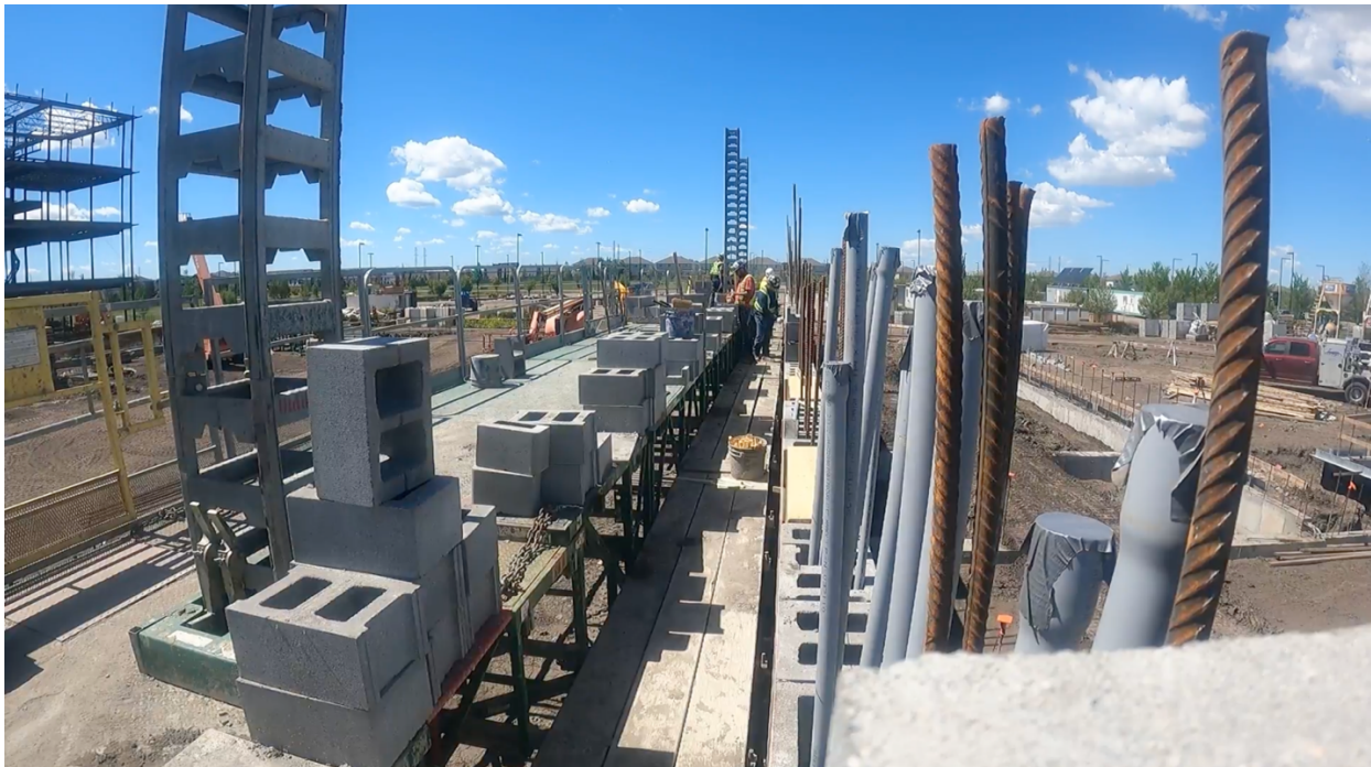
Figure 11: Mortar and CMU blocks Stations
