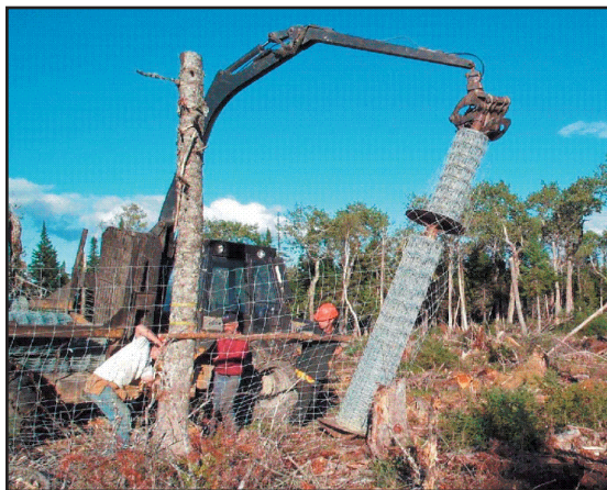
Figure 2 a): Construction of fences around the mosaic of cutblocks. Photo courtesy of Produits forestiers Anticosti Inc.
