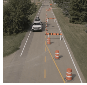
(b) Example of work zone image.
