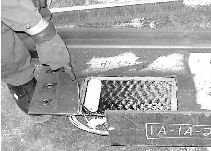
Figure 3-12 Application of FRP patch to steel beam
