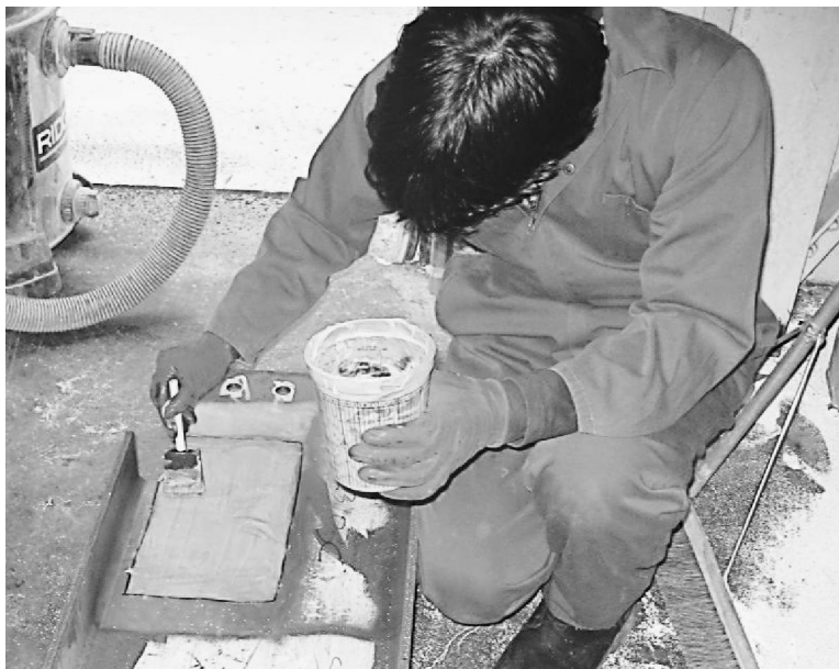
Figure 3-10 Application of Sikadur® 330 primer to SHL3103C
