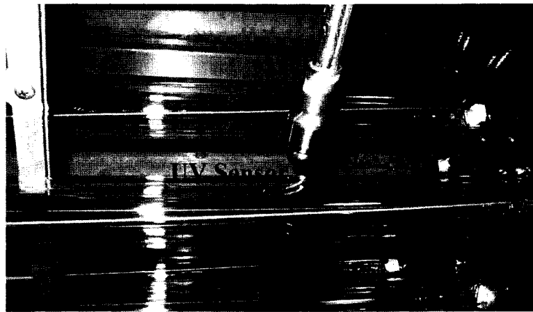
Figure 6: UV Sensor placed in Alberta Capital Region WWTP UV Reactor
