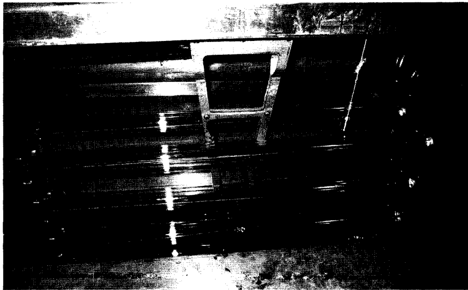
Figure 16: UV Module consisting of a dual (side-by-side) row configuration of UV lamp assemblies
