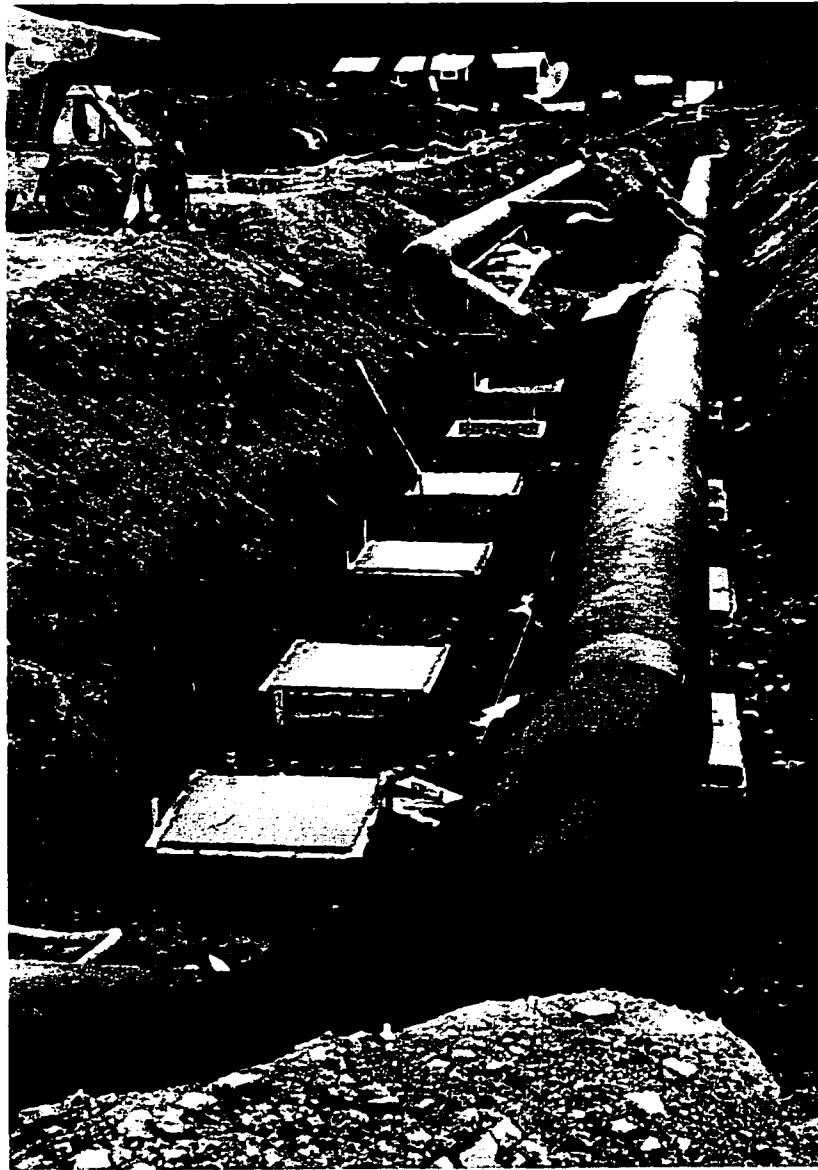
Figure 1.1 Typical sleeper-supported pipe installation
