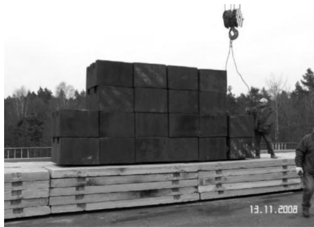
Figure 2.5. Concrete slabs and steel blocks used for proof load testing (Olaszek et al., 2010)
