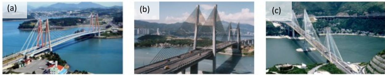
Figure 2.9. (a) Jindo Bridge, (b) Kap Shui Mun Bridge, (c) Ting Kau Bridge (Jang et al., 2010) (Wong, 2004)
