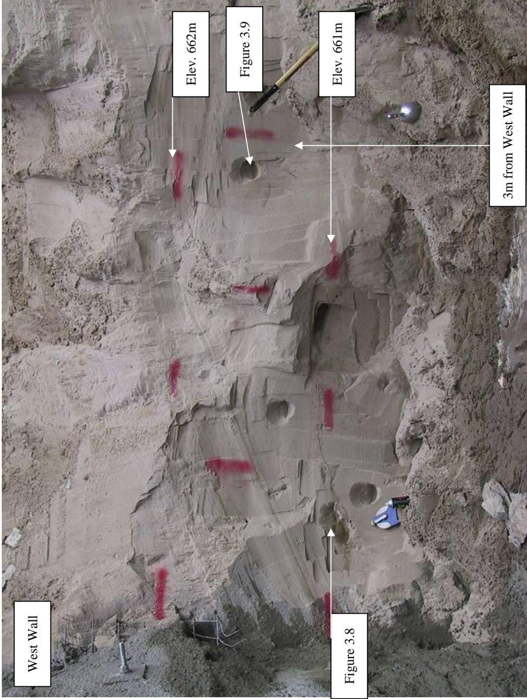
Figure 3-6 Mapping of exposed face of Outwash Sands and Silts during portal excavation, south facing along West Wall
