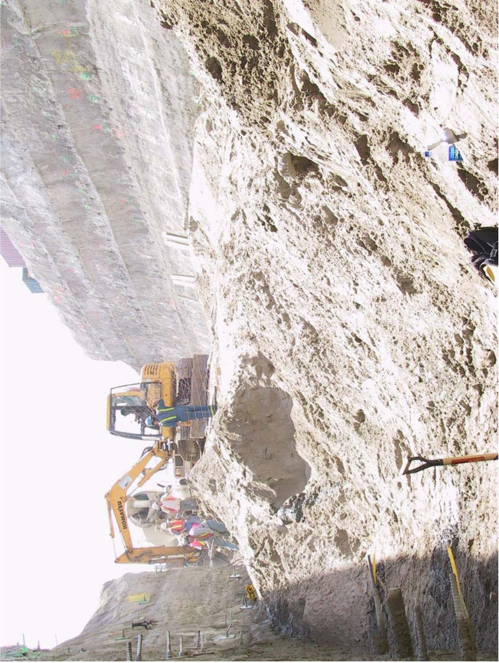
Figure 3-5 Edmonton SLRT portal near end of excavation, within the Outwash Sands and Silts – May 23, 2003.
