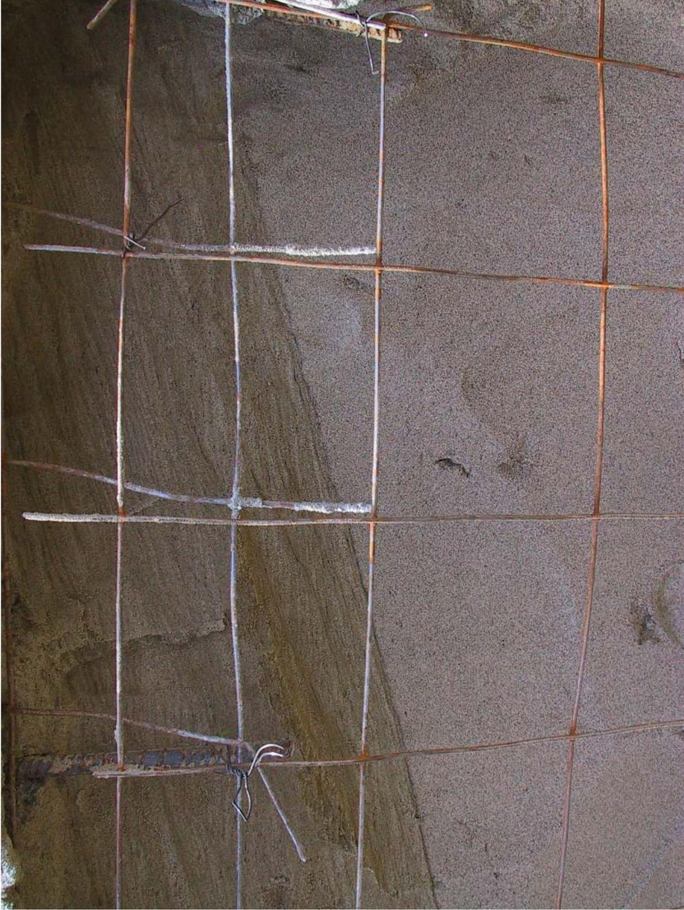
Figure 3-14 Transition from clean sand to sand with silt stringers (elev. 666m).
