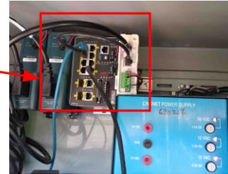
(e) Cable communication between RSE and controller via the additional switch device
