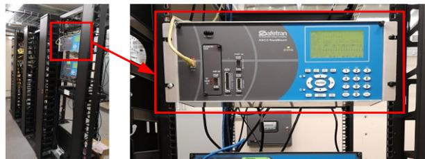
(e) Cable communication between RSE and controller via the additional switch device
