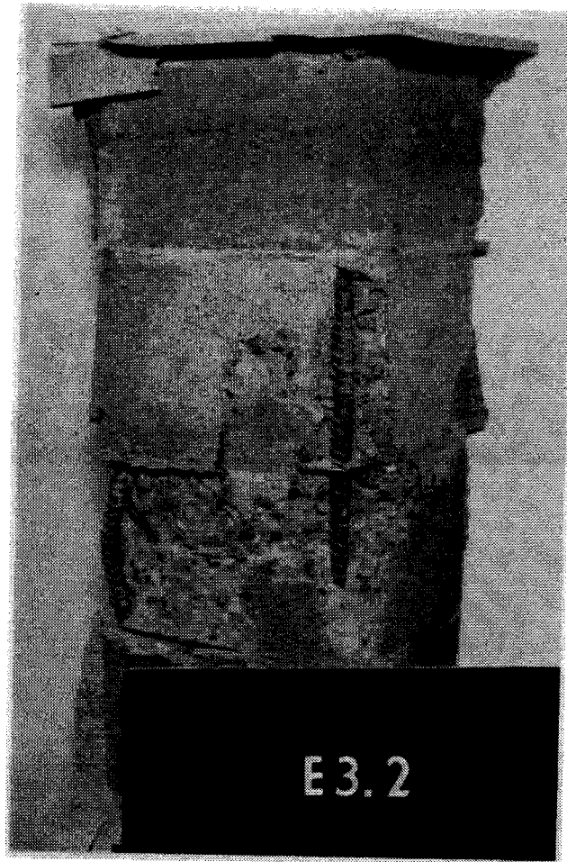
PLATES 5.24, 5.25, and 5.26 Type 1 Eccentrically Loaded Column Failures
