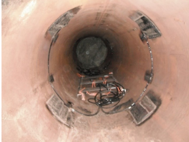
Figure 5.2. Strain gauges installed inside the pipe
