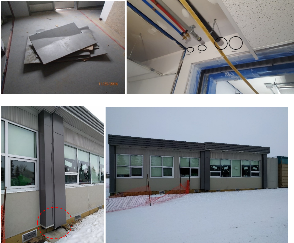
Figure A- 12. Problems and challenges regarding connecting the modules
