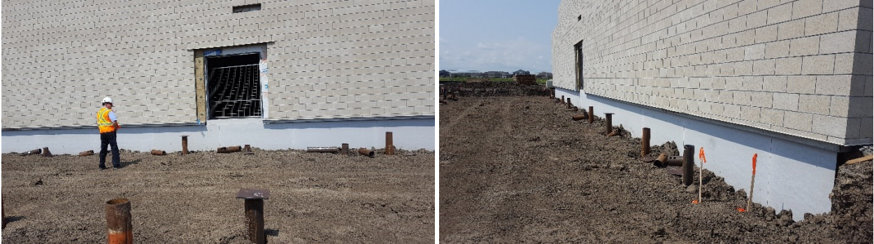
Figure A- 1. Installation of foundation piles
