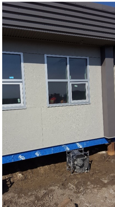
Figure A- 16.Flooding should be dried before starting the work
