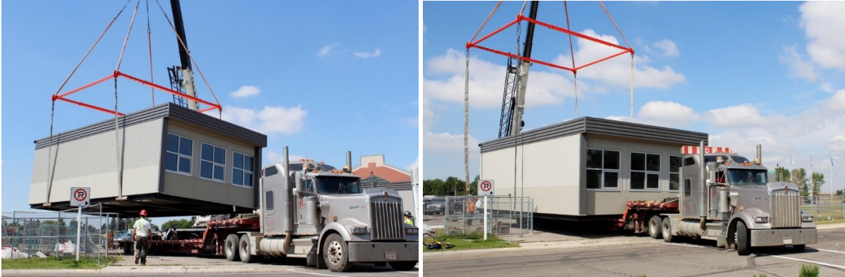
Figure A- 2. The positioning of modular classrooms using cranes (Palliser 2019)
