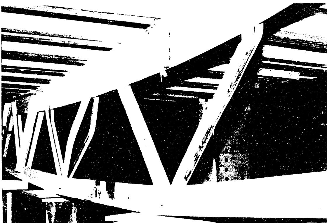
Fig. 9.11 Bottom chord after truss failure (no load)
