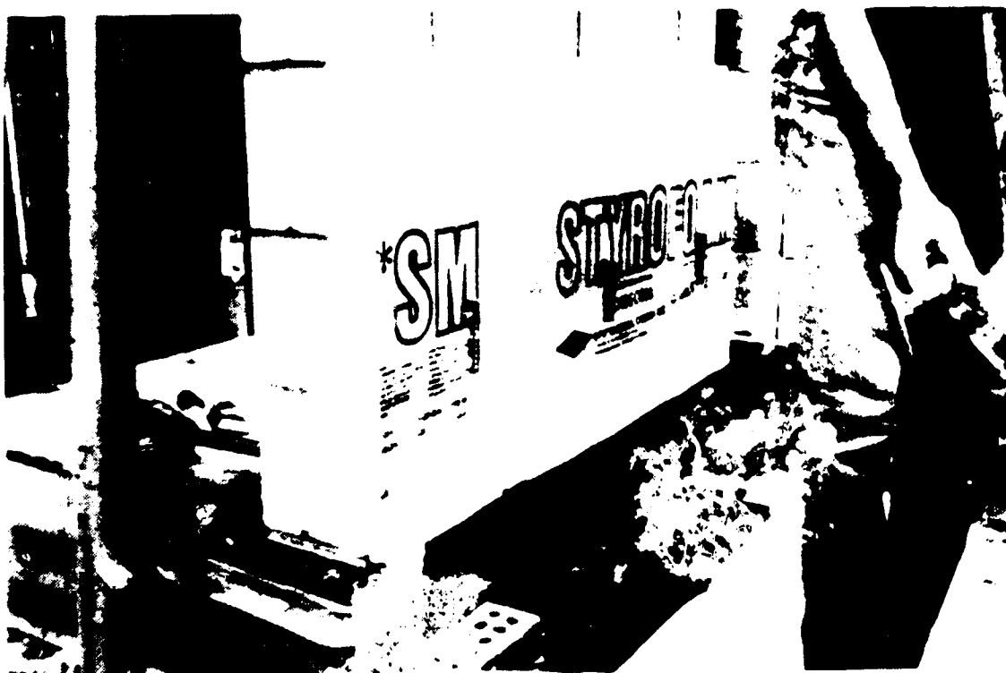
Plate 5.6 Application of Insulation to Block Wythe
