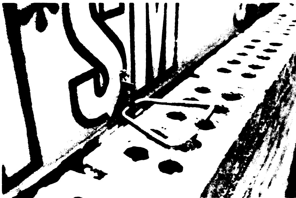
Plate 3.2 Detail of Connection of Shear Connector-Veneer Construction
