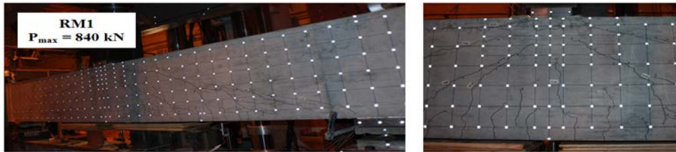
b) Crack Patterns after Failure
