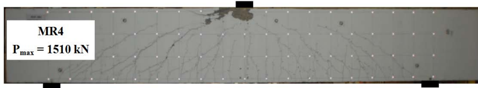
b) Crack Patterns after Failure
