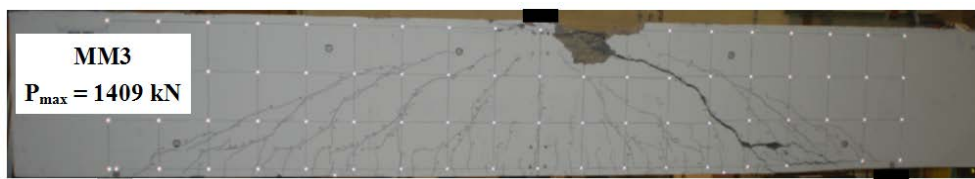
b) Crack Patterns after Failure
