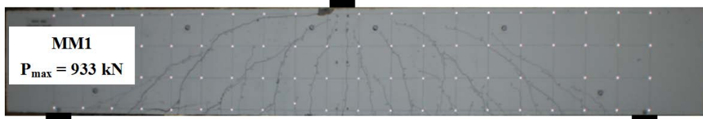
b) Crack Patterns after Failure
