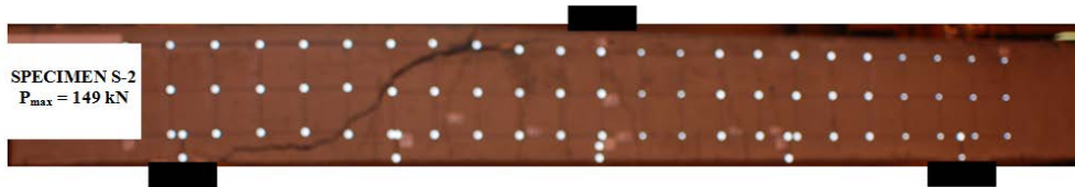
d) Crack Patterns after Failure
