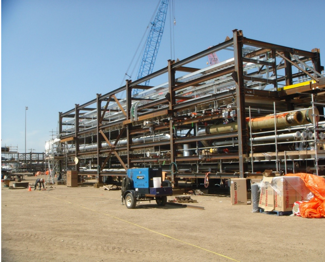
Figure 1-1 a typical pipe-rack module
