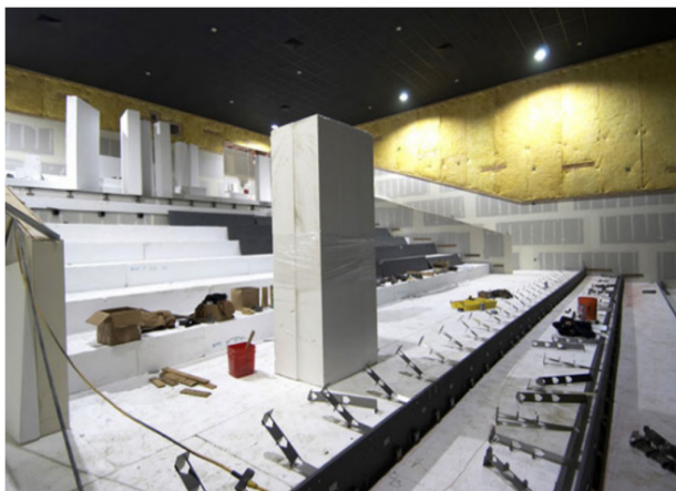
Figure 2- 8: Applications of EPS geofoam: a) buried pipelines; b) abutment backfill; c) stadium and theatre seating; d) roadway construction (EPS Industry Alliance 2012).
