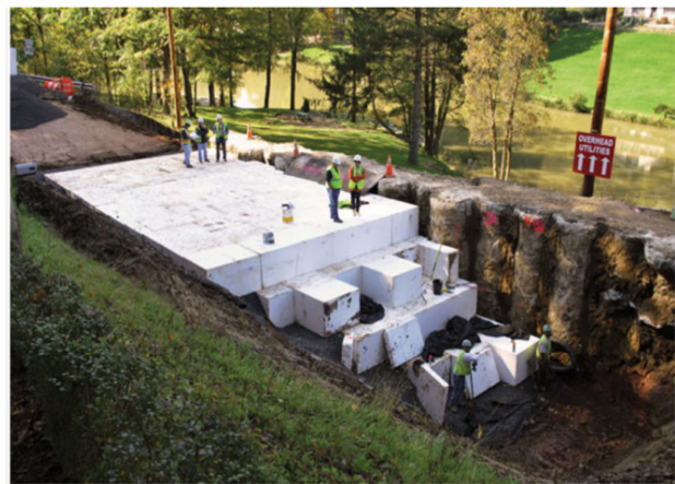
Figure 2- 8: Applications of EPS geofoam: a) buried pipelines; b) abutment backfill; c) stadium and theatre seating; d) roadway construction (EPS Industry Alliance 2012).
