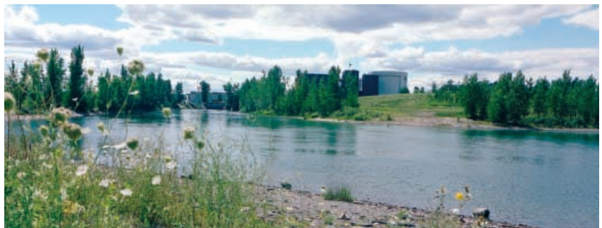
Gentilly-2 nuclear generating station
