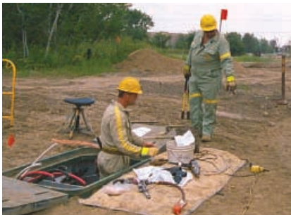
Distribution system undergrounding
