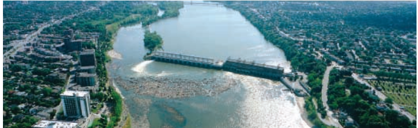
Rivière-des-Prairies generating station
