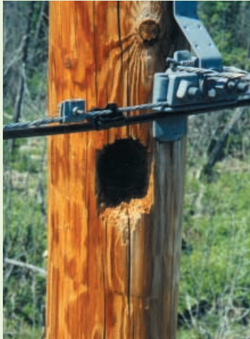
Pole damaged by woodpeckers
