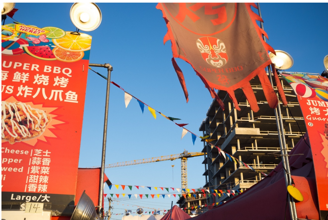
Figure 9 - New construction around the night market, August 4, 2018.
