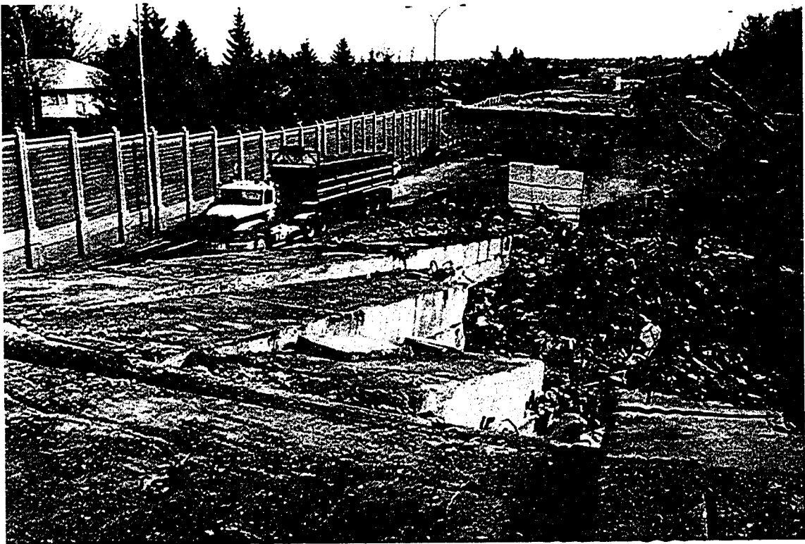
Photo 3.1: Old Crowchild Trail Bridge Superstructure under Demolition
