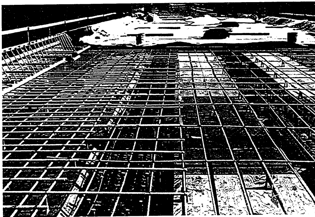
Photo 3.5: Reinforcement in Negative Moment Region
