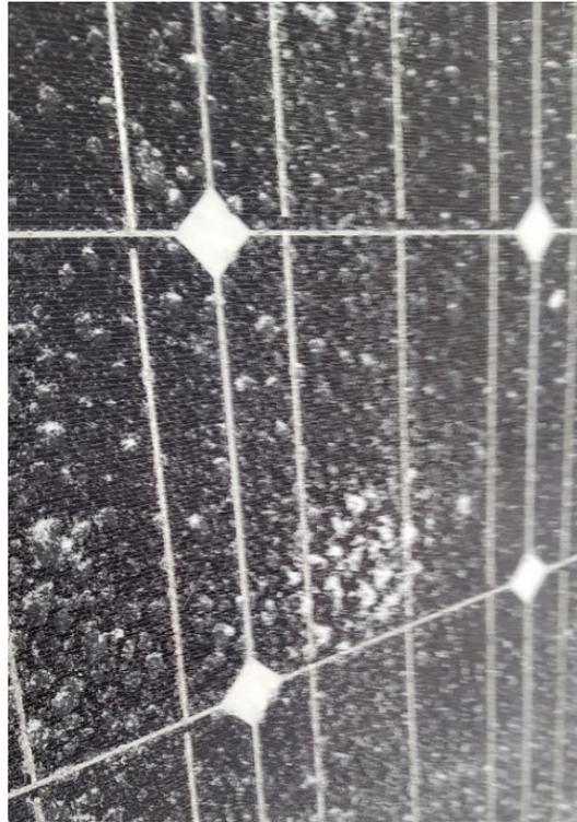
*Figure 4.2 Ice on the framed PV resulting from snow melting on contact (Event 1)*
