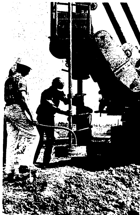
FIGURE: 4.11 LOAD CELL BEING LOWERED INTO THE HOLE.
