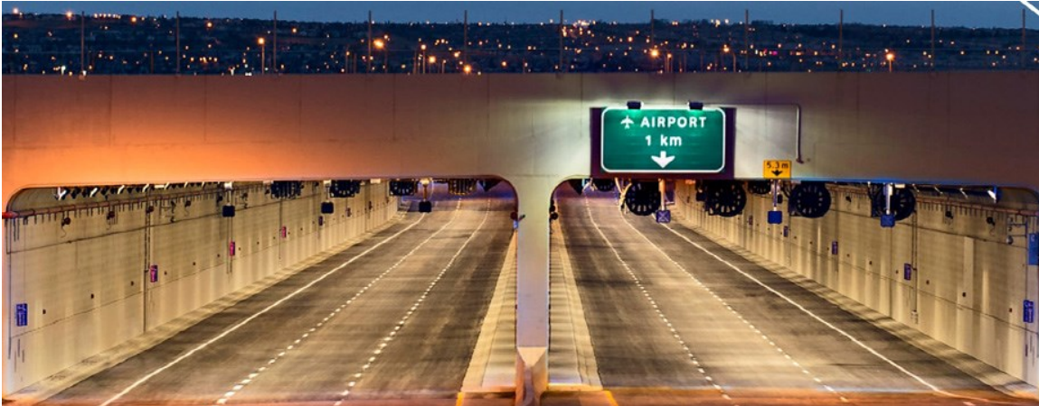
Figure 3.4 Calgary Airport Trail Tunnel looking East (Associate Engineering, 2016)
