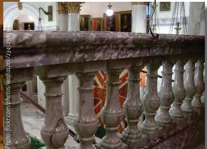
Marble finish to column and balustrades in the Rotunda
