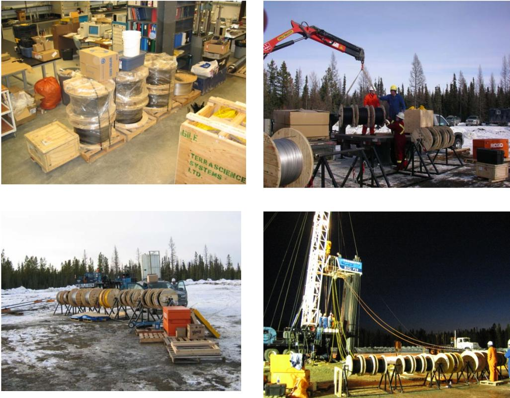
*Figure 4.5 Top Left: Spool and instrumentation prepared for transport to well site. Top Right: Unloading and assembling the spools and cable for instrumentation. Bottom Left: All instrumentation and spools ready for running the cables over the sheaves. Bottom Right: View of the cables passing over the sheaves during night-time [17].*
