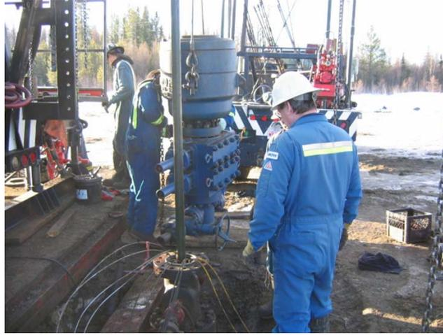
Figure 4.8 Cables passing through the dognut after removal of the blowout preventer (blue).
