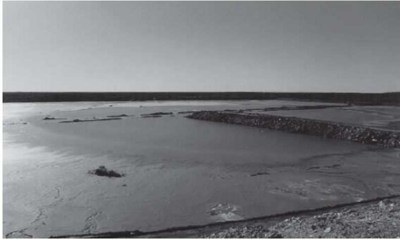
Figure 2.3 Typical saline gold tailings storage in arid region, Western Australia (Newson and Fahey, 2003).
