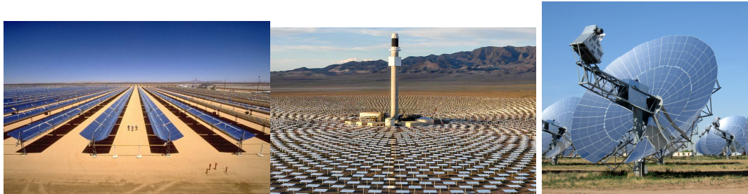
Figure 1.3. The parabolic trough power plant in California (left), a solar power tower in Nevada (center), and a solar dish concentrator (right). Images taken from Ref. 23
