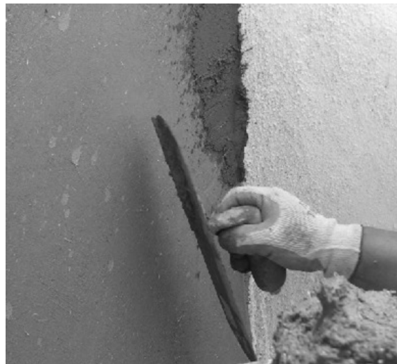
Figure 3.8: Surface after application of joint compound.
