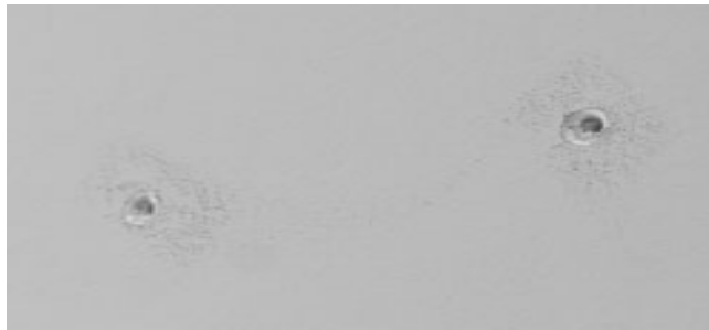
Figure 4.18: Nails in drywall
