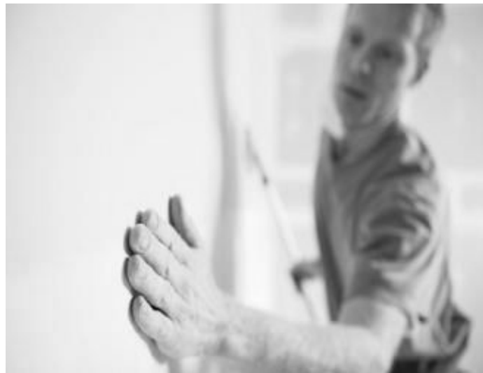
Figure 2.5: Manual process of assessing surface smoothness.
