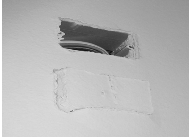
Figure 3.7: Dry Wall surface with an electric socket hole and mudded area
