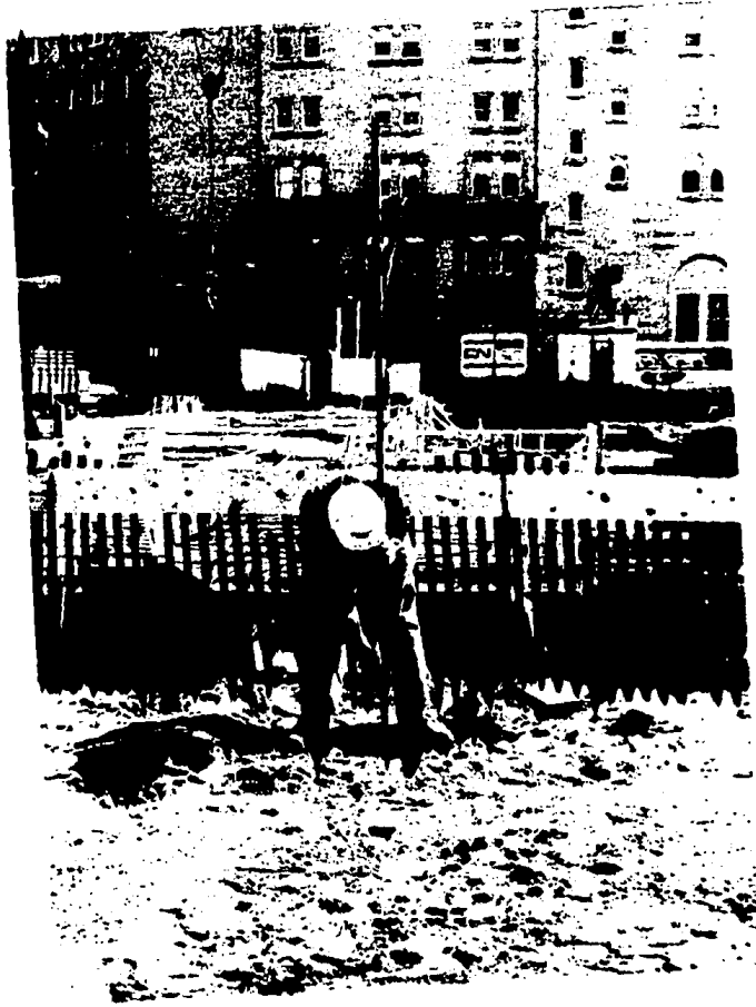
FIG. 5.11 REPROBING PROCEDURE AT GROUND SURFACE
