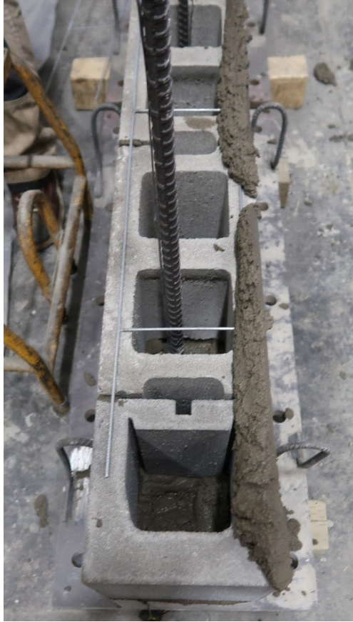
Figure 3.6 – Specimen Construction (Bed Joint Reinforcement)
