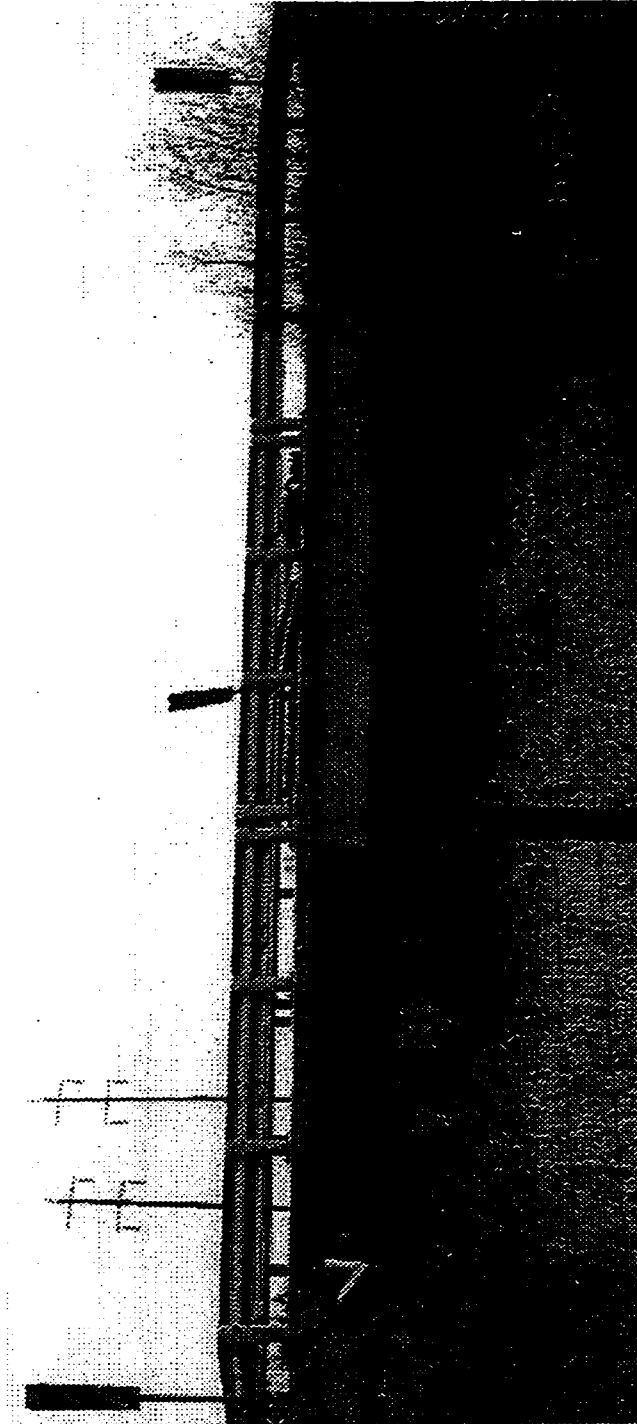
Fig. 4.1 Photo of Clearwater Creek Bridge with CFRP Sheets on 1 Span
