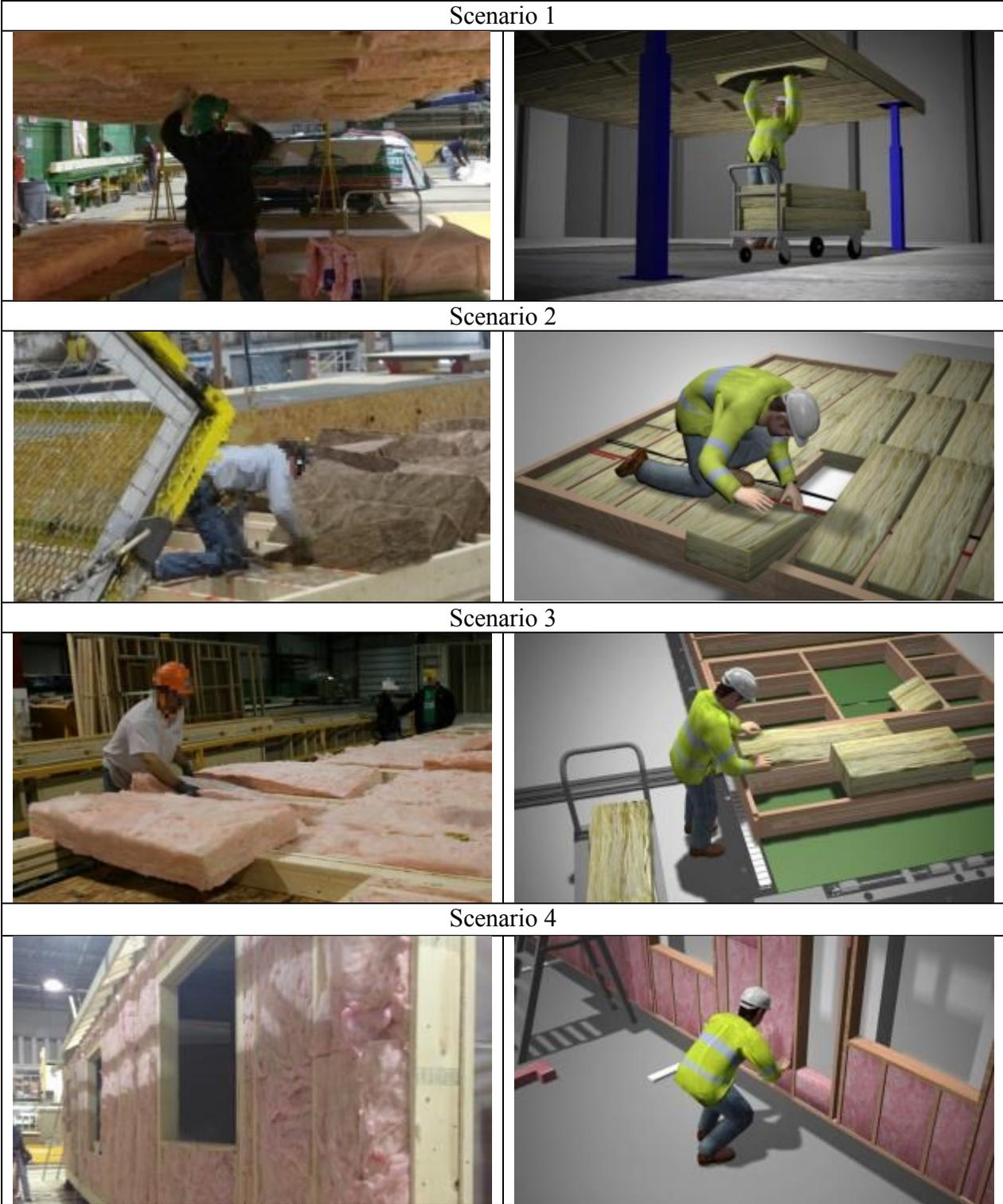
Figure 5.9: Four scenarios for placing insulation
