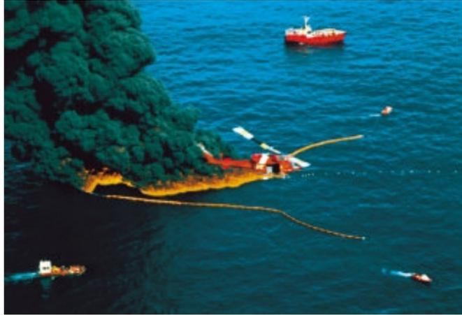
**Figure 1.4** In-situ burning methodology to remove an oil spill from the water surface.[1]
