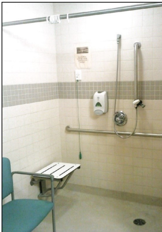
Figure 4.20. Roll-in shower stall with flip-down bench seat. Shelving was lacking for patients to store their own shampoo, conditioner, body wash, and towels, all items that therapists were teaching them how to use for independent self-care.
