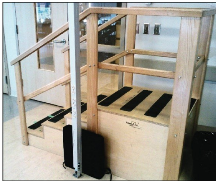
Figure 4.23. Stairs in the physio gym.
