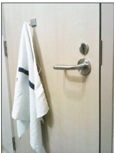
Figure 4.19. Towel hanging on the shower room door. Towels were relatively small (22 x 42 inches) towel hooks were positioned to be accessible from a wheelchair.
