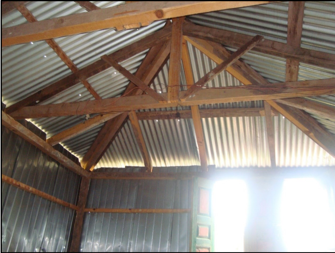
Figure 1-7: Traditional wooden roof structure in Langarpura.
