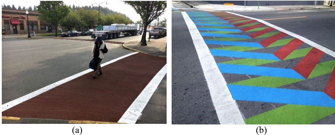
Figure 3.9: Example of crosswalks with (a) effective colour contrast for people with dementia (Chew, 2017), and (b) undesirable pattern (Design TAXI Crew, 2017)
