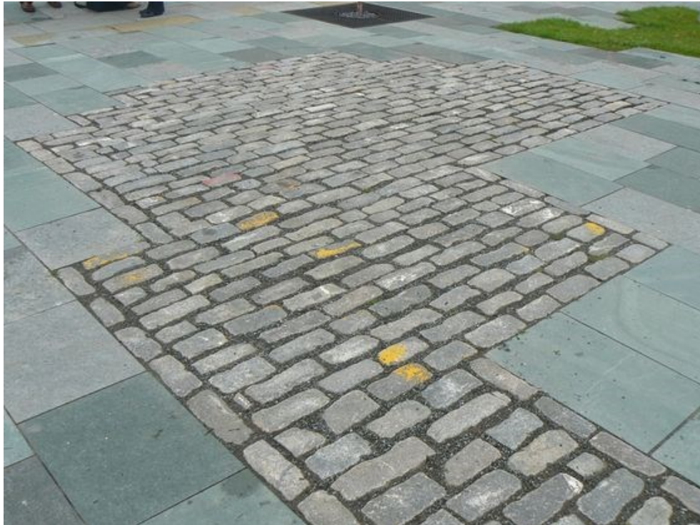
Figure 3.11: Example of hierarchical paving (Ced Stone Group, 2017)
