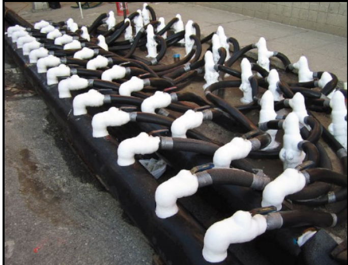
Figure 18: Mass artificial ground freezing
