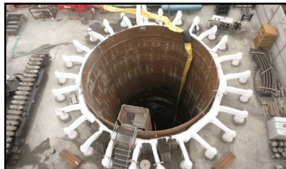
Figure 17: Peripheral artificial ground freezing
