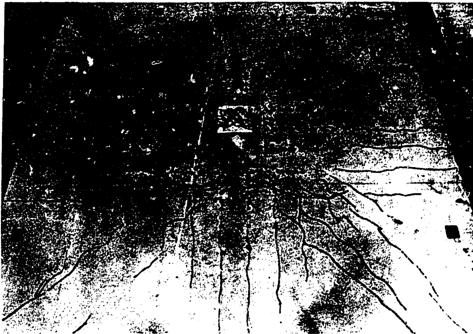
Figure 4.20 Top Crack Pattern: P19RC
