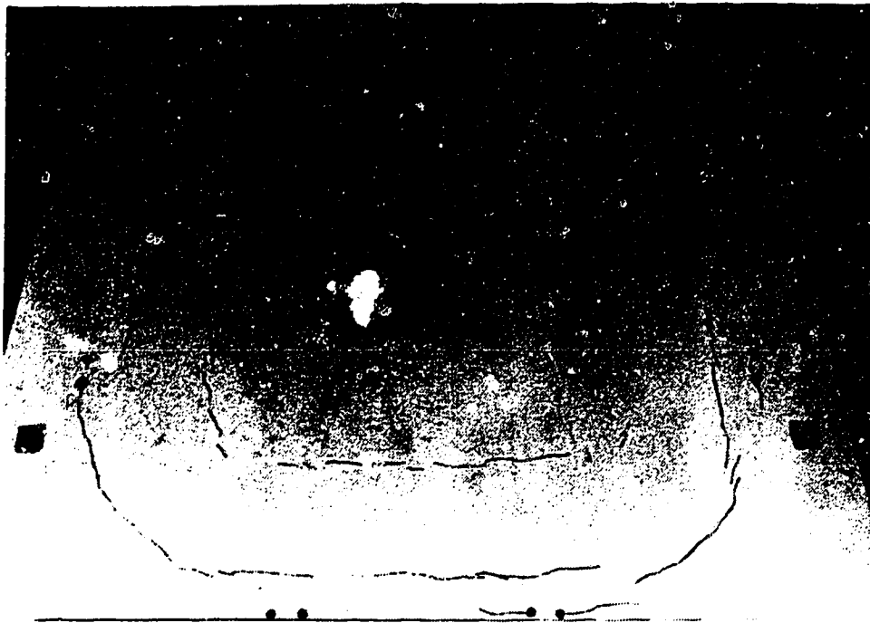
Figure 4.21 Bottom Crack Pattern: P19RE
