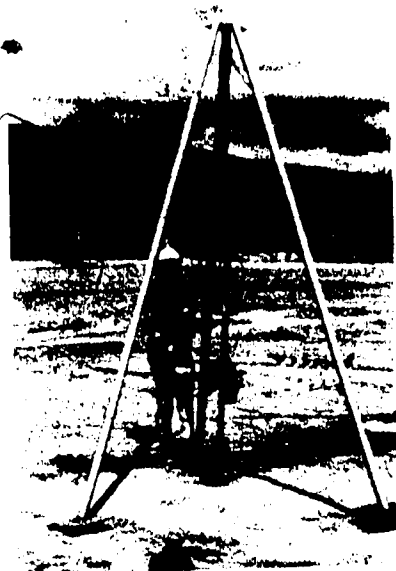
Figure 4.19 Tripod and drop hammer arrangement
