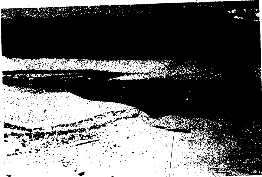
Figure 7.4 Photograph illustrating water accumulation on otherwise clean sand during sand placement by hydraulic fill method.
