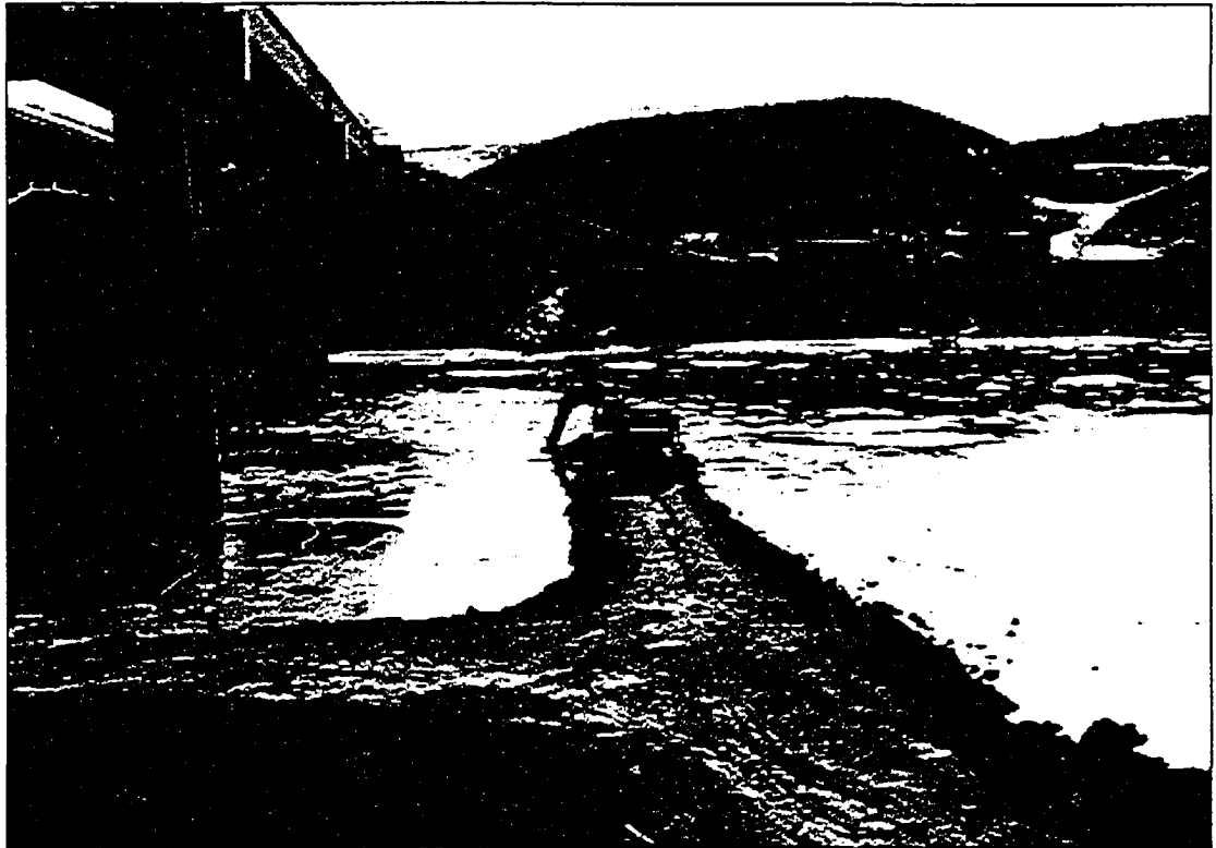
Figure 4.11. Case history project on the North Saskatchewan River in Edmonton, Alberta, west berm removal, March 2001.
