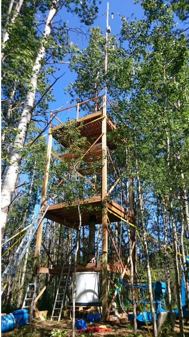
Figure 3.A. 1. Wooden structure supporting the focus tree after the cut. The focus tree is placed in the white bucket resting on the scale. Taken the 12 th of July 2017, in Thorhild County, AB, Canada.
