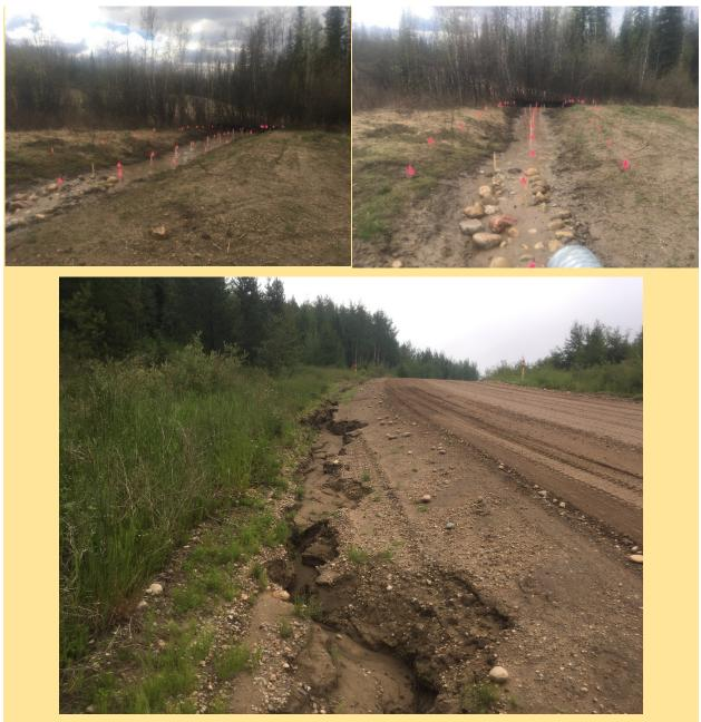
Figure A14. P4108 plot photos (clockwise from top left): (1) Oblique view of plot set up with centreline and boundary flags, and labelled silt marker stakes. (2) Centerline view of plot. (3) Section of road downslope of plot prior to fence installation. Culvert failure in 2016 or earlier caused rilling of the ditchline and deposition of a major plume at the road drain point.
