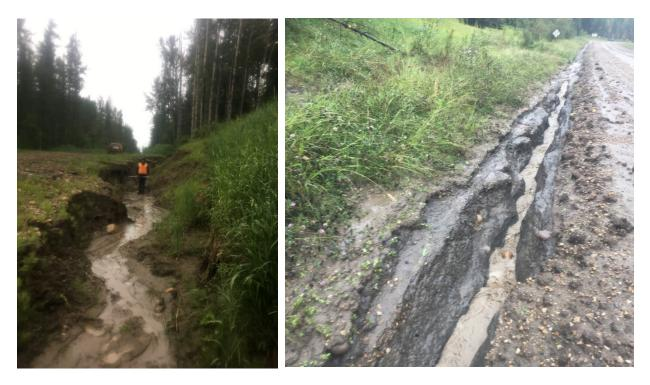
Figure 5-3. Channelized ditch erosion in the Simonette. Deep erosion with partial undermining of the road prism (left), long, narrow, and deep channel depositing in Deep Valley Creek (right).
