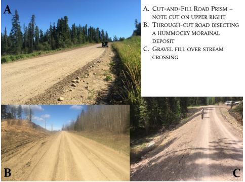
Figure 1-3. Examples of different types of road cut and fill.
