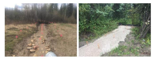
**Figure 2-3. Typical silt fence erosion plots in the Simonette** *The left shows a silt fence under dry conditions, the right shows ponding during a rain event.*
