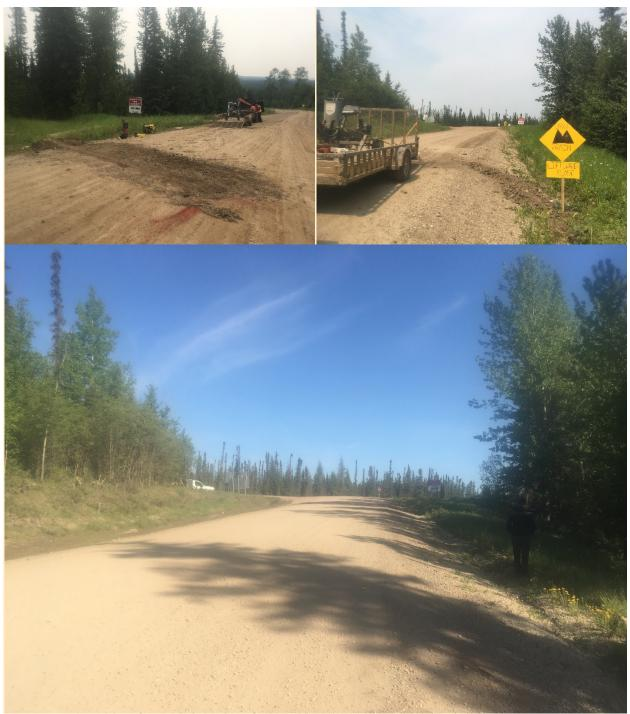
Figure A3. P4107B pictures of road surface: (top left) upper culvert installation, (top right) bottom of plot, (bottom) overview of road showing thick, well-gravelled fill
