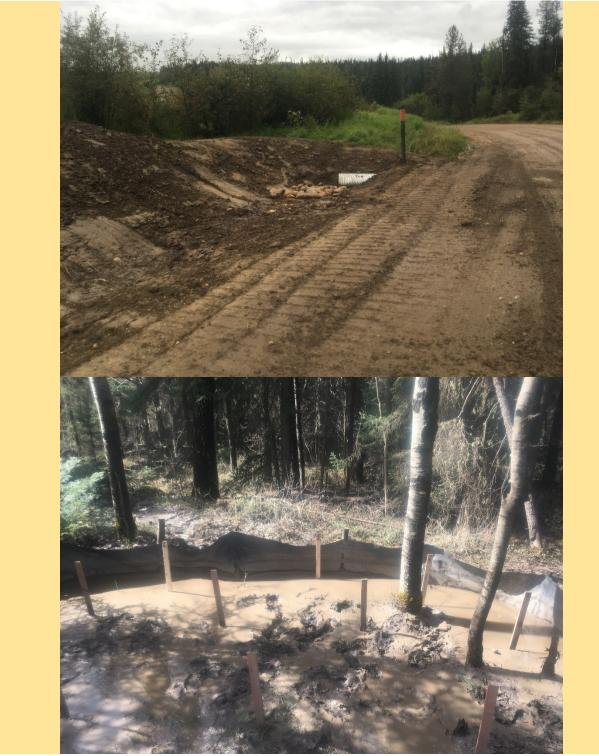
Figure Al6. Site photos of P4106. Top: Repaired culvert with rocks around intake (rocks are also at the outlet). Bottom: Silt fence with thin mud layer after a storm. While there was some deposition at the site, it was very difficult to measure with the stakes, probably not more than 0.5-1cm.
