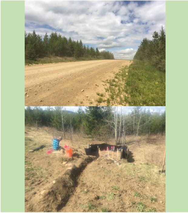
Figure A17. Site photos of P4126. Site was installed in a low-gradient (2.5°) segment of road (top), and a turnout berm was hand-excavated just up-gradient of a previous settling location with some sediment in it (bottom). Overall low slope and possible bypass may have compromised the ability of this plot to produce a meaningful sediment signature.
