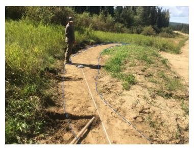
Figure 3-1. A plume or road sediment deposited in an excavated roadside turnout
