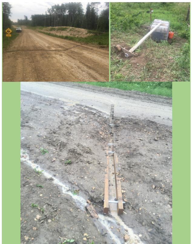
Figure A10. P7131 site photos, road with steel trough culvert, showing worn clay surface (top left), settling tank intake (top right), road surface in wet conditions showing plastic deformation.
