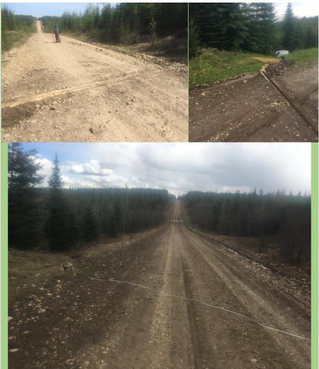
Figure All. P4128 site photos, freshly-installed top culvert in dry conditions showing mixed stony soil with silt (top left), lower plot boundary after rain (top right), marked lower plot boundary in spring in moist soil conditions (bottom).
