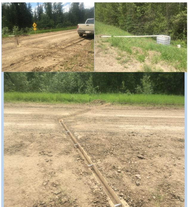
Figure A6. M270 culvert bounding lower edge of plot (upper left); settling tank (upper right); detail of road surface showing gravel mixed in with silty fill material (bottom).
