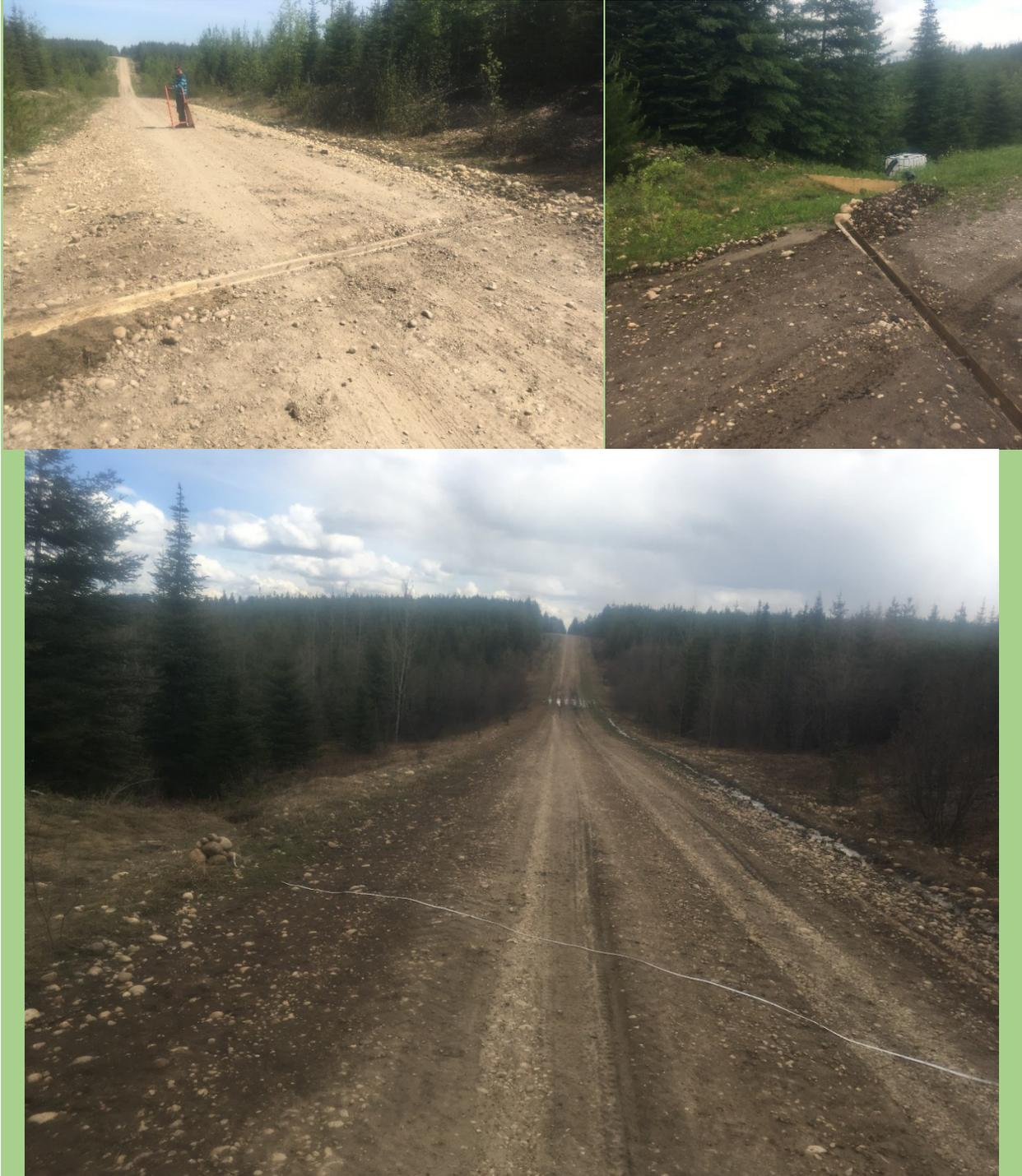
**Figure A11. P4128 site photos, freshly-installed top culvert in dry conditions showing mixed stony soil with silt (top left), lower plot boundary after rain (top right), marked lower plot boundary in spring in moist soil conditions (bottom).**
