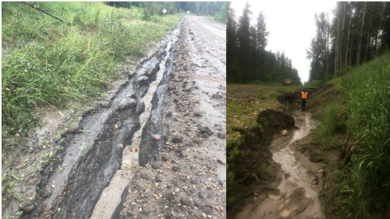
**Figure 1-5. Severe gully erosion in ditches, Simonette watershed, Alberta.**
