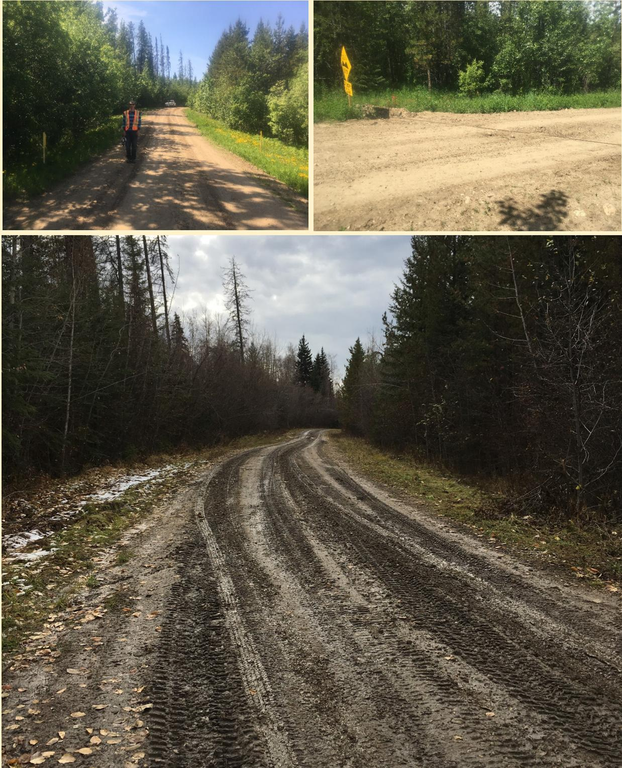
**Figure A5. Pictures of P295, bare plot (upper left), plot with culvert installed (upper right), road site in saturated fall conditions, showing intrusion of underlying fine-grained material (bottom).**
