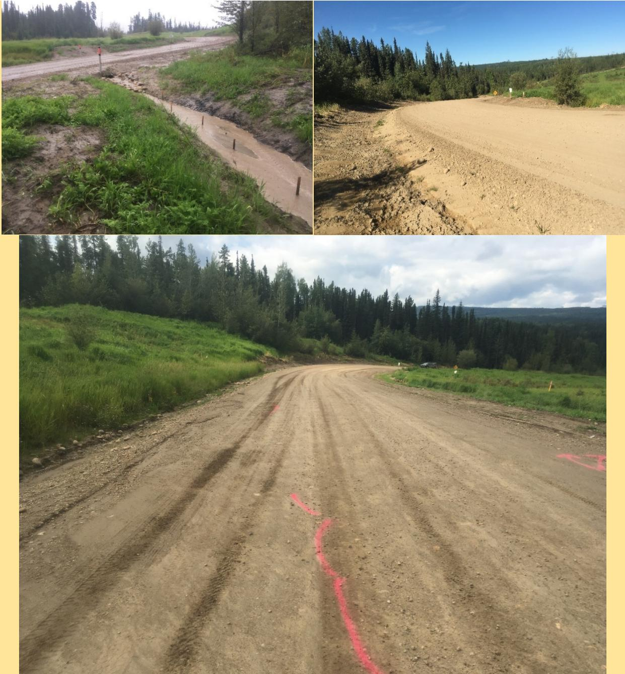
**Figure A13. Photos of P4107 silt fence plot, from top left: outflow of culvert in front of settling fence (out of view), road in dry conditions, well-gravelled sandy road surface after a summer rainstorm.**
