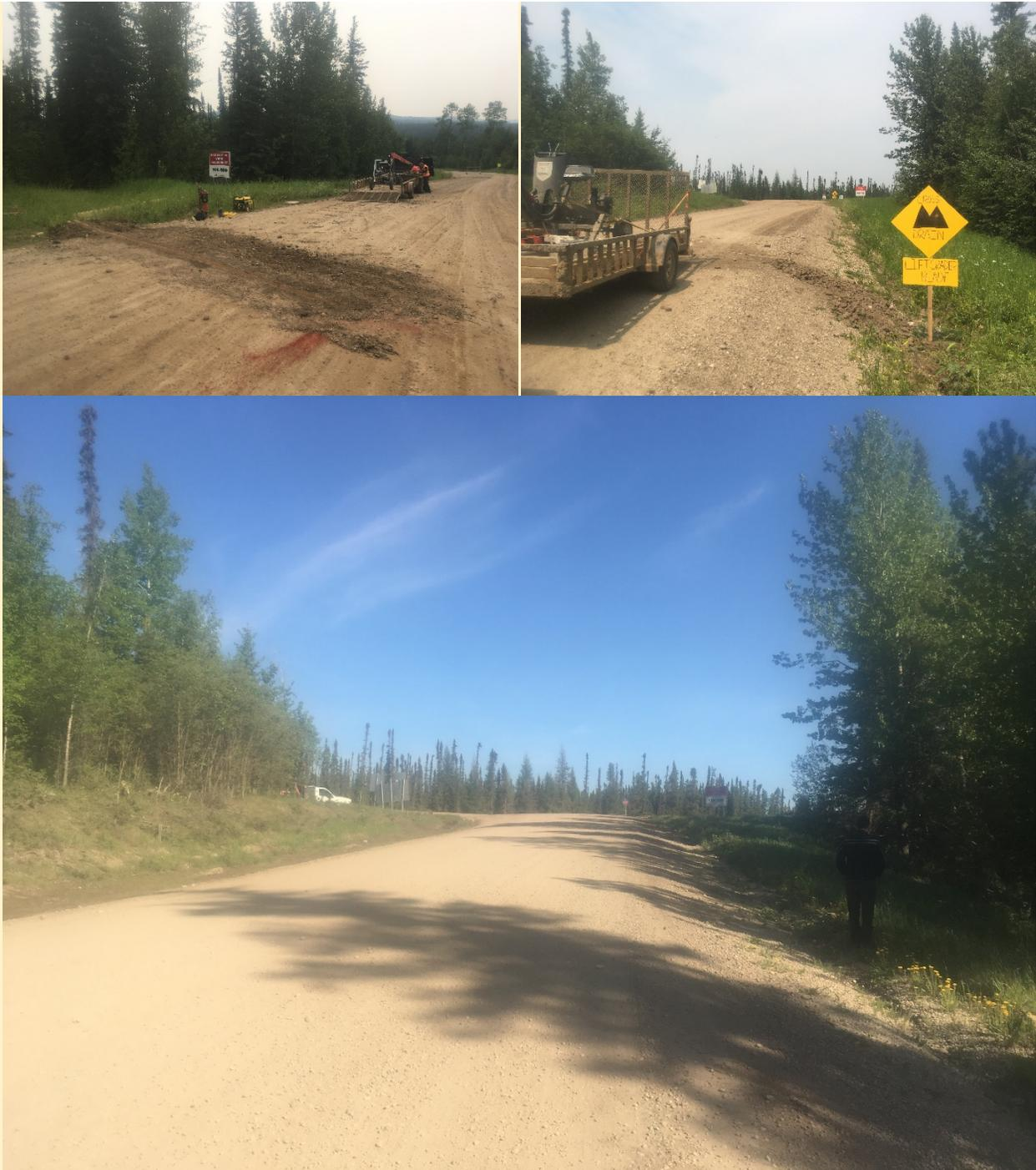
**Figure A3. P4107B pictures of road surface: (top left) upper culvert installation, (top right) bottom of plot, (bottom) overview of road showing thick, well-gravelled fill**
