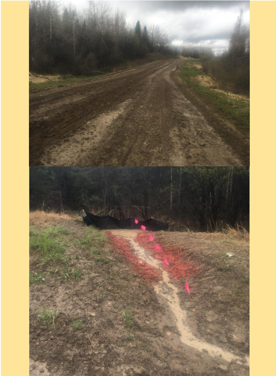
**Figure A15. P4111 Site Photos: (top) looking downslope from P4111 drain point. Road has more silty material in this area and nearby soil pits are clayey luvisols with an illuviated clay hardpan. Plot outlet (bottom) showing flagging and plot delineation. This was a relatively small plot overall.**
