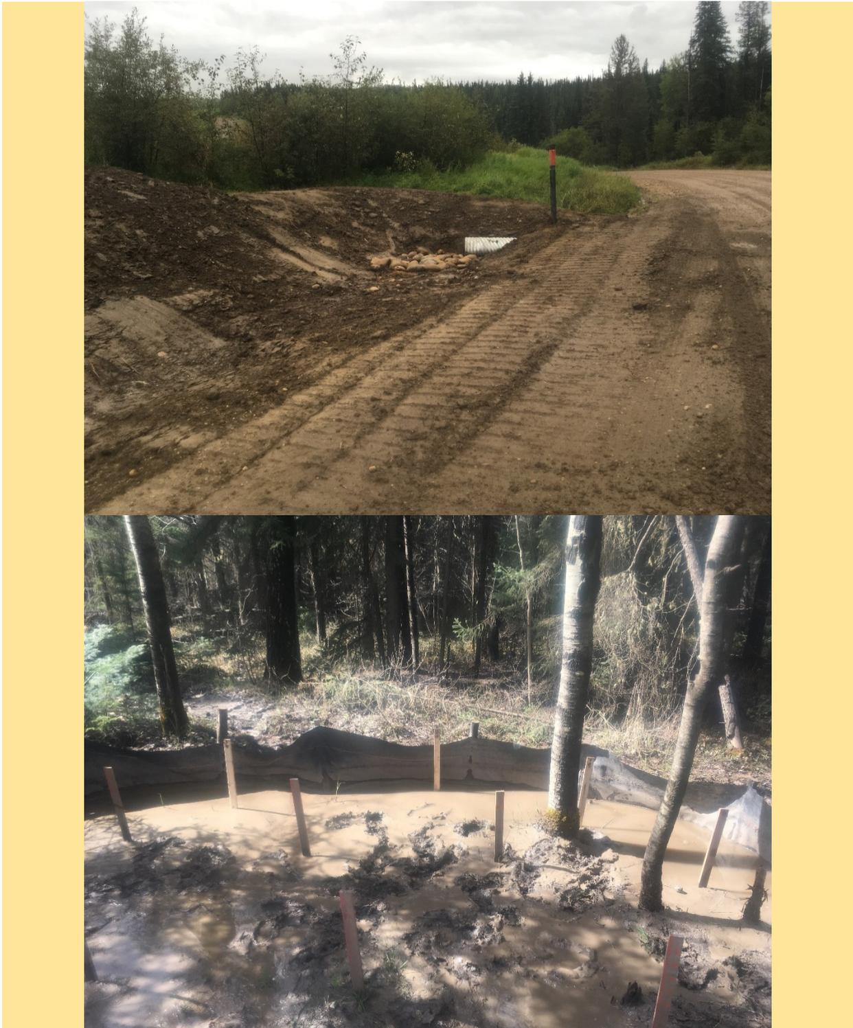
**Figure A16. Site photos of P4106. Top: Repaired culvert with rocks around intake (rocks are also at the outlet). Bottom: Silt fence with thin mud layer after a storm. While there was some deposition at the site, it was very difficult to measure with the stakes, probably not more than 0.5-1cm.**
