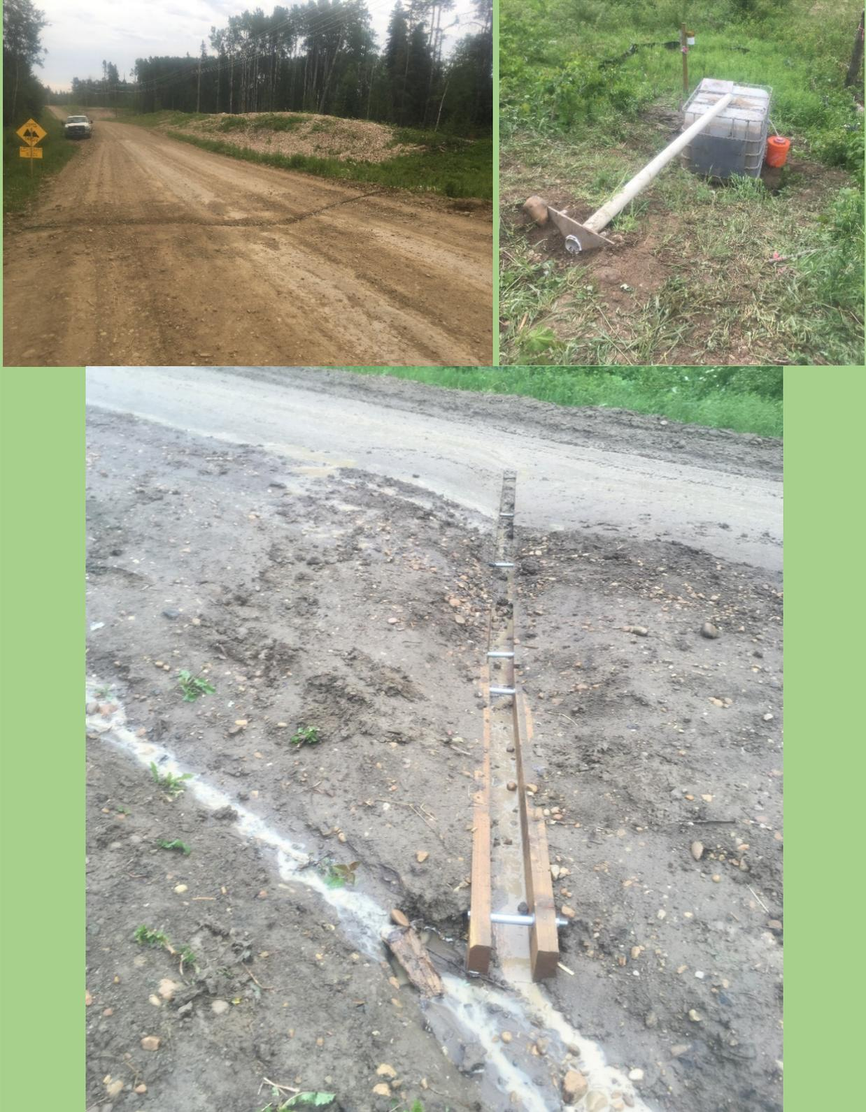
**Figure A10. P7B1 site photos, road with steel trough culvert, showing worn clay surface (top left), settling tank intake (top right), road surface in wet conditions showing plastic deformation.**
