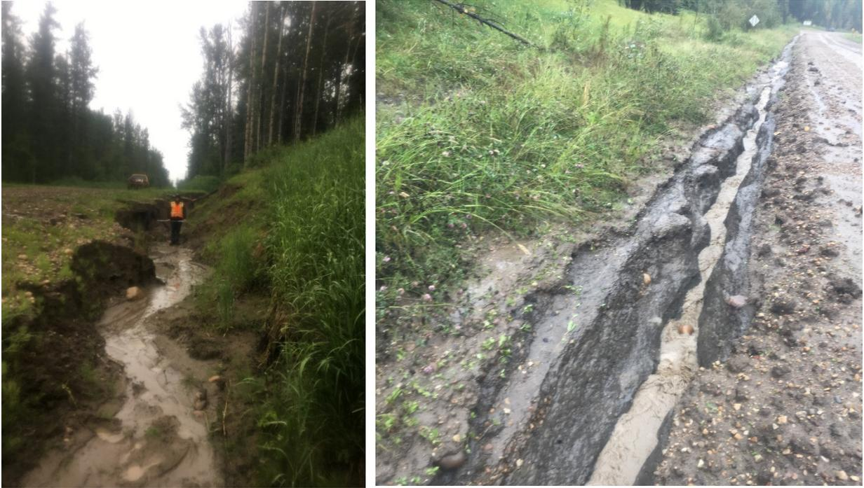
**Figure 5-3. Channelized ditch erosion in the Simonette. Deep erosion with partial undermining of the road prism (left), long, narrow, and deep channel depositing in Deep Valley Creek (right).**
