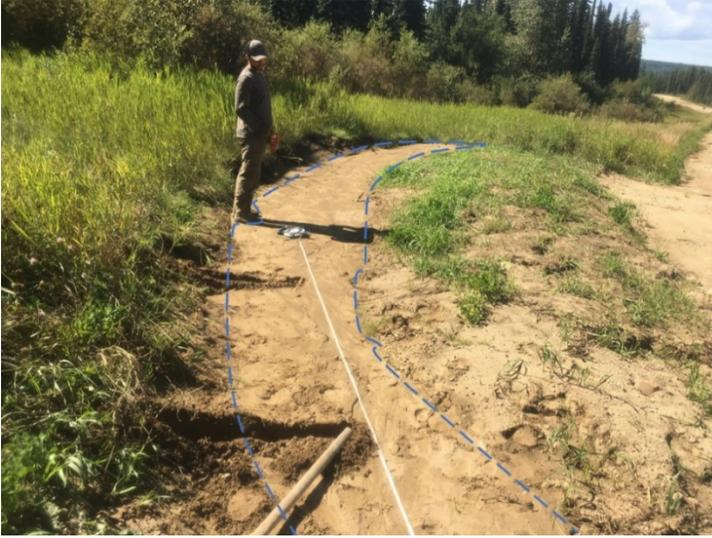
Figure 3-1. A plume or road sediment deposited in an excavated roadside turnout
