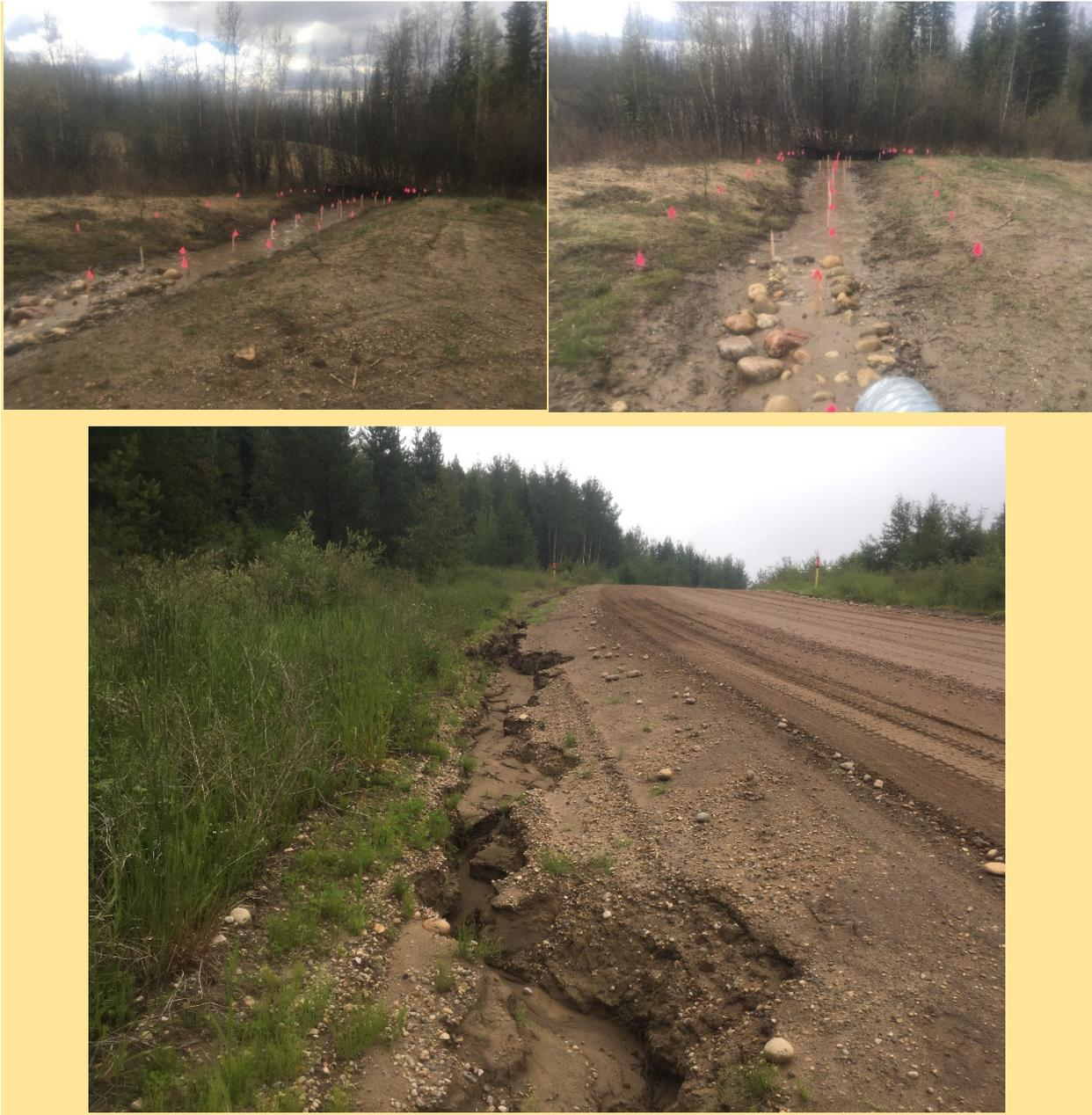
**Figure A14. P4108 plot photos (clockwise from top left): (1) Oblique view of plot set up with centreline and boundary flags, and labelled silt marker stakes. (2) Centerline view of plot. (3) Section of road downslope of plot prior to fence installation. Culvert failure in 2016 or earlier caused rilling of the ditchline and deposition of a major plume at the road drain point.**
