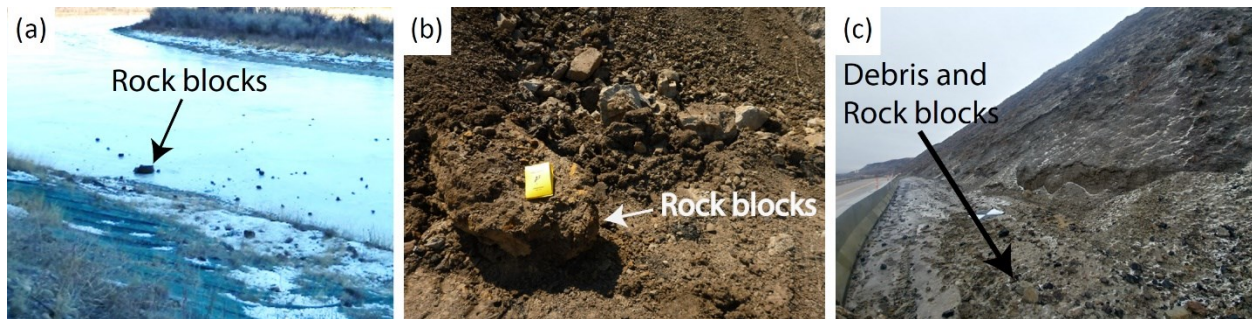
Figure 3-3 Slope failures at the C018 slope; (a) rock blocks found on the frozen Red Deer River on December 2017; (b) rock blocks found across the Highway on May 2018; (c) accumulation rock falls and debris slide behind jersey barrier on November 2018.
