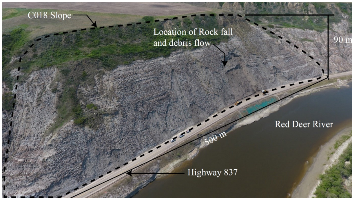
Figure 1-1 Photograph of the C018 slope taken by UAV inspection following a slope failure on May 23, 2018 (Klohn Crippen Berger 2018a).
