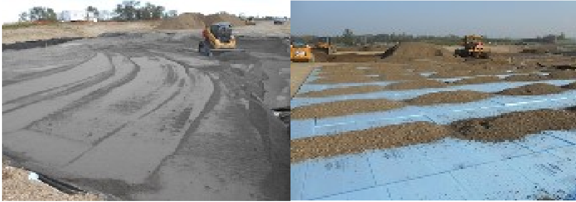
Figure 3-1: Placement of the (left) Bottom ash and polystyrene boards (right)
