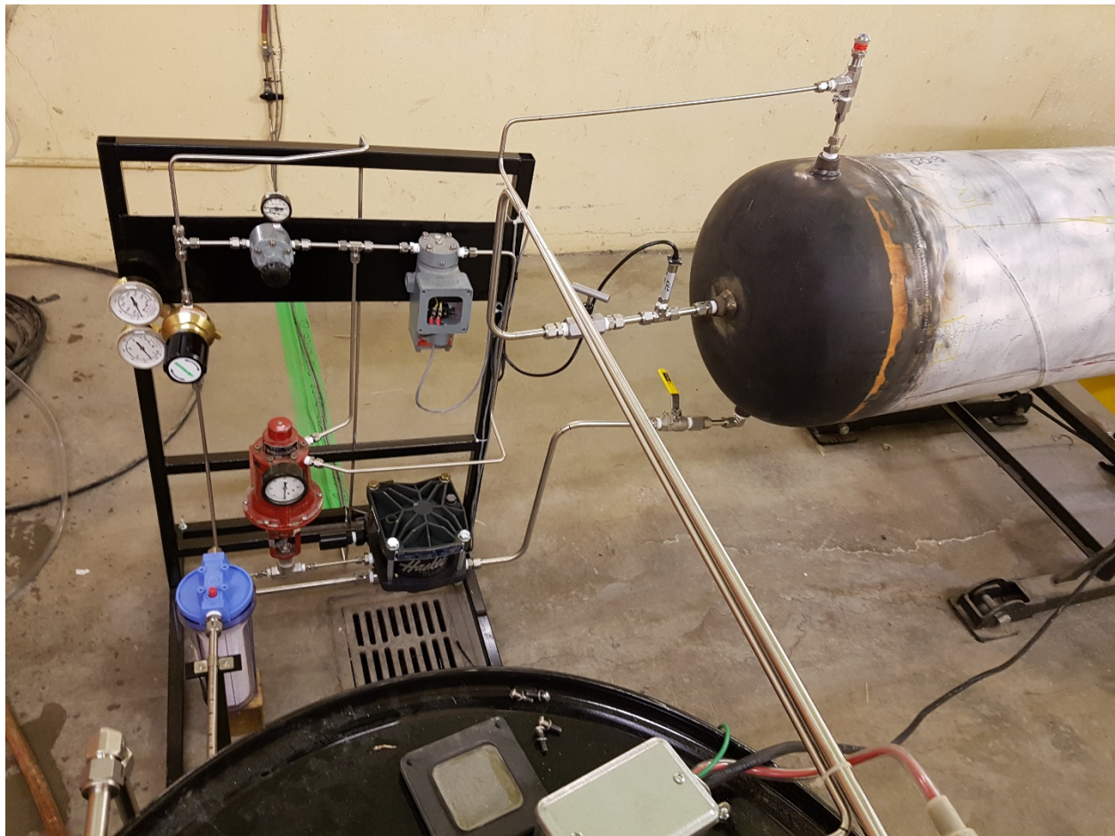
Figure 3.8 Photograph of the plumbing system built for the full-scale test.
